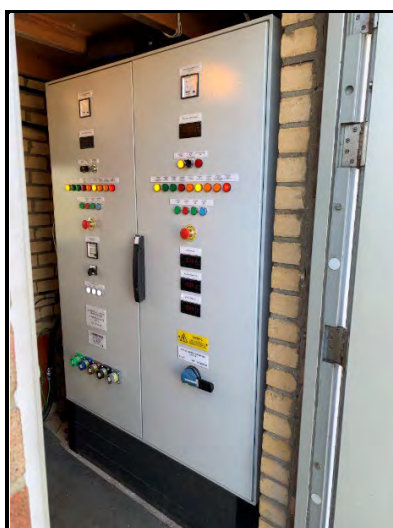
New switchgear at Sutton Bridge Sluice – installed March 2025
