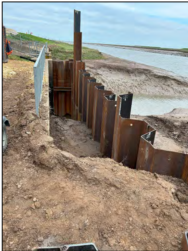
Views of the installation of the new sheet piling forming the southern tidal wingwall
