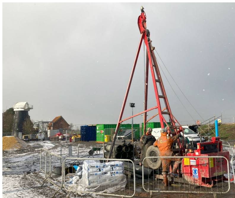
Installation of temporary de-watering well using shell and auger rig.
