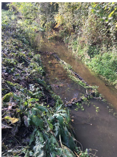
Coir matting with plants pegged in the Lamsey Beck, Eye, behind the log flow deflectors.
