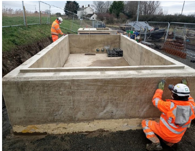
Control kiosk base. Finished floor level will be at the top of the concrete.
