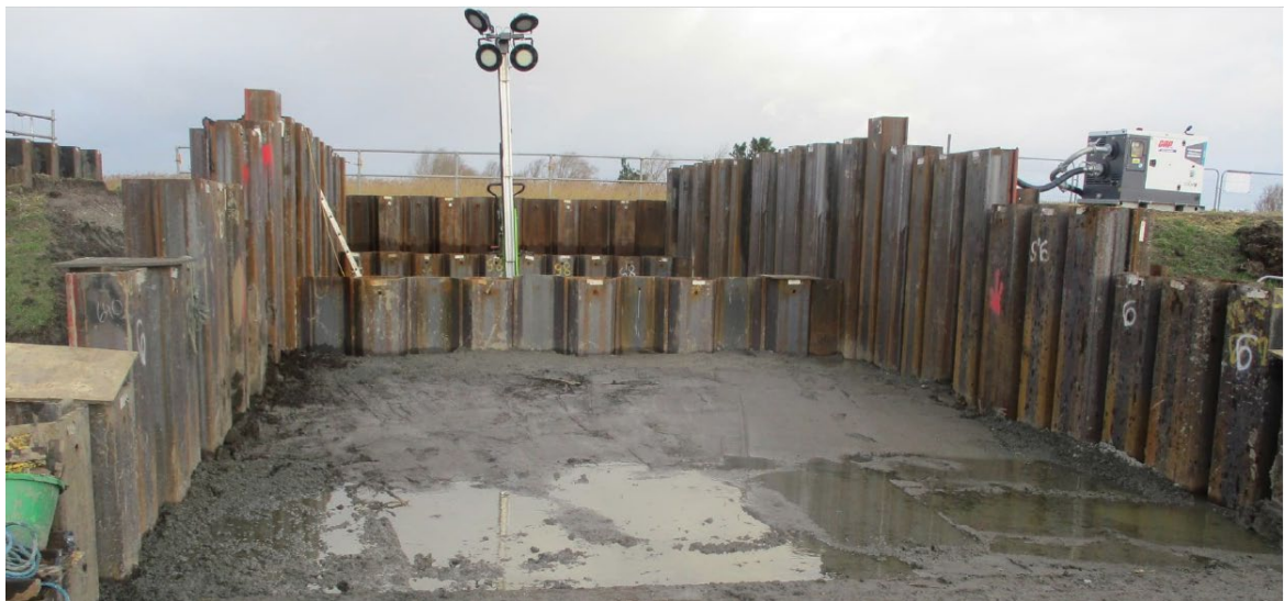
Completed pumping station piling viewed from the inlet.
