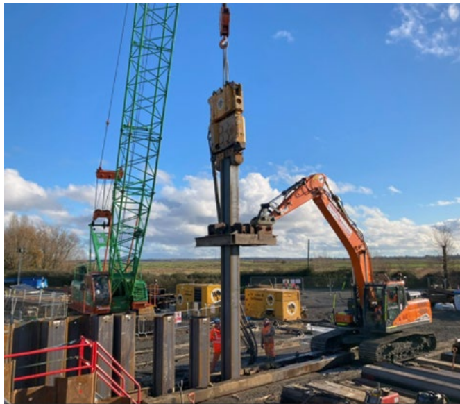
Piles being installed using a suspended vibro hammer.
