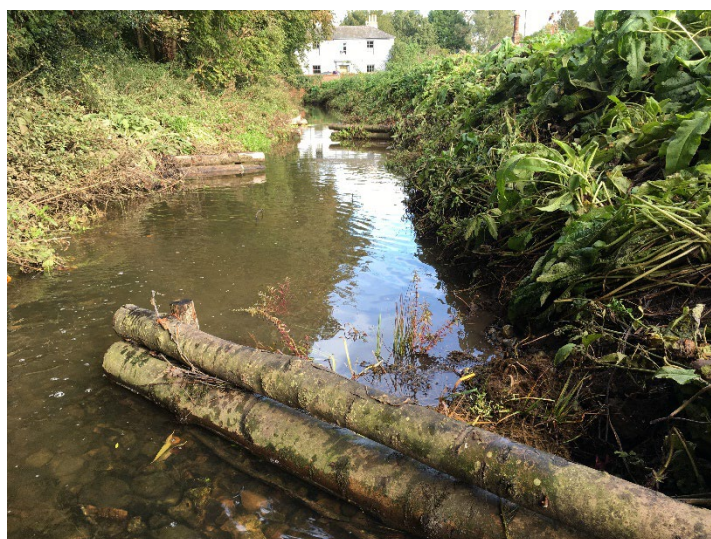
Coir matting with plants pegged in the Lamsey Beck, Eye, behind the log flow deflectors.
