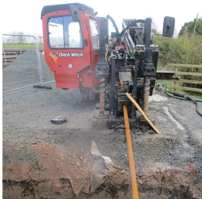
Directional drilling rig installing cable ducts for electric cable under IDB main drain.
