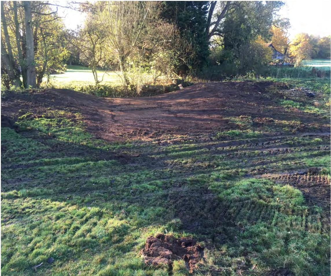
Bank lowering in isolated locations to activate the floodplain quicker during high level events
