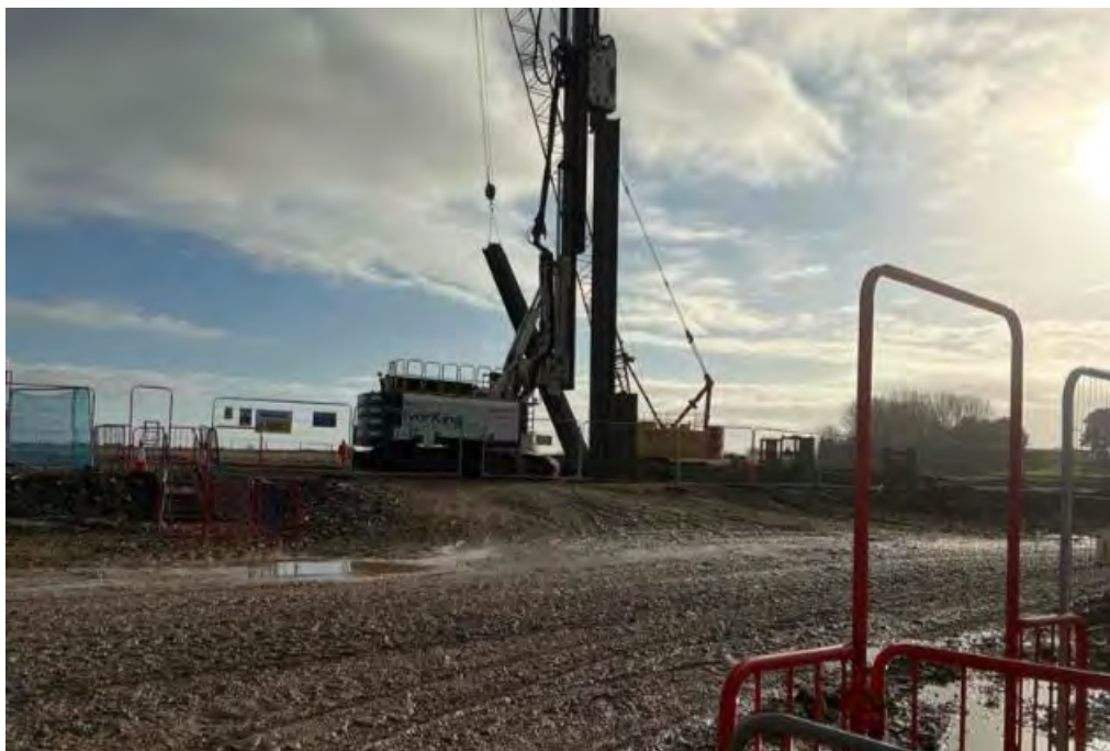
Sheet Piling at Lothingland PS, mid-January
