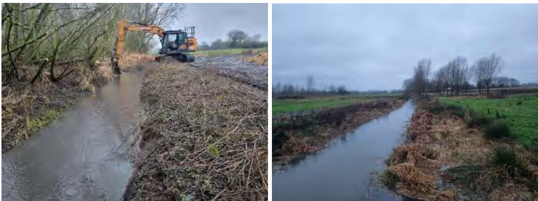
2050m of desilt and vegetation removal completed.
