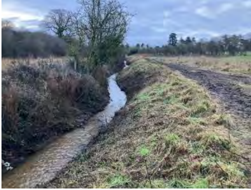
De-silt and vegetation management completed.
