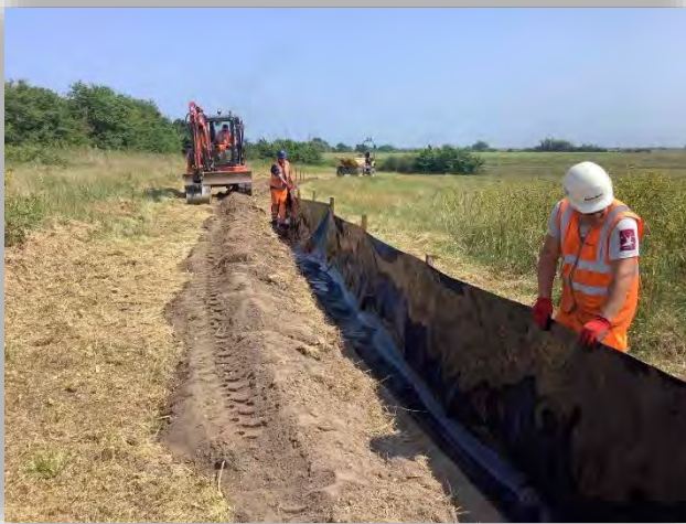
Reptile Trapping Fence Installation
