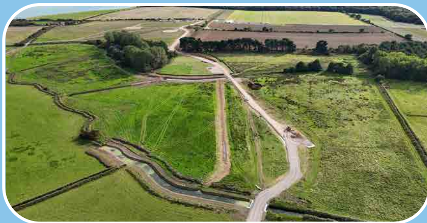
Above: The temporary haul route, established to support efficient material movement across the valley, allowing clay imports to be positioned to build the new flood embankment
