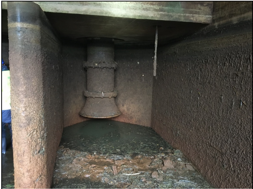
Fleet Haven pump sump – view of one of the existing bell mouths – Nov 2019
