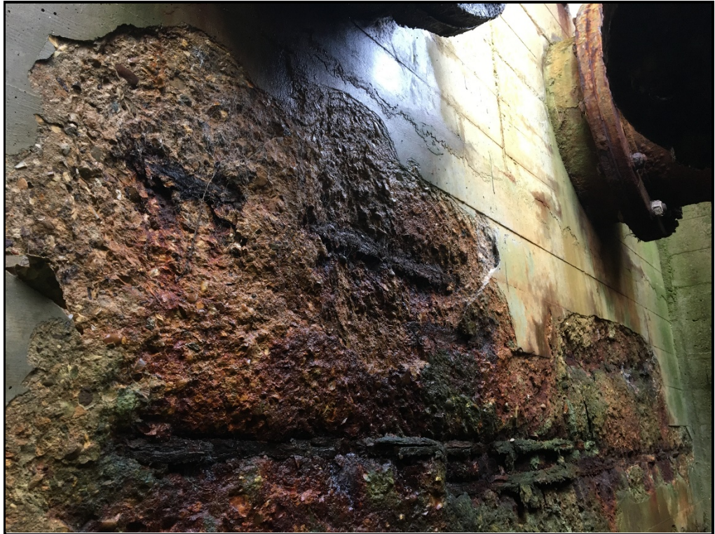
Fleet Haven surge chamber – view of some of the concrete damage showing exposed, badly corroded reinforcing bar – Nov 2019
