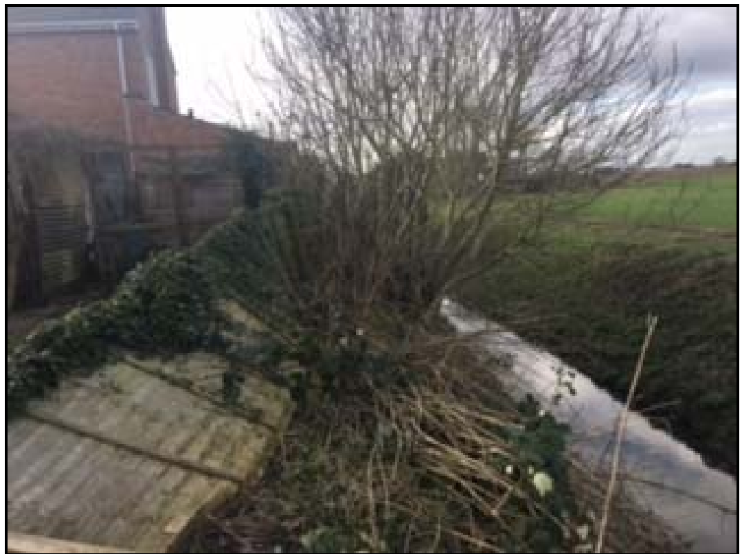
Photograph showing Board's Old Peartree Drain on right, remains of old boundary fence on drain brink, and end of existing garage on far left.
