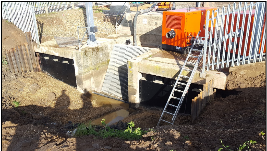
Sheet piling works completed – painted and concrete infill in place. View prior to bank re-forming and removal of dam.
