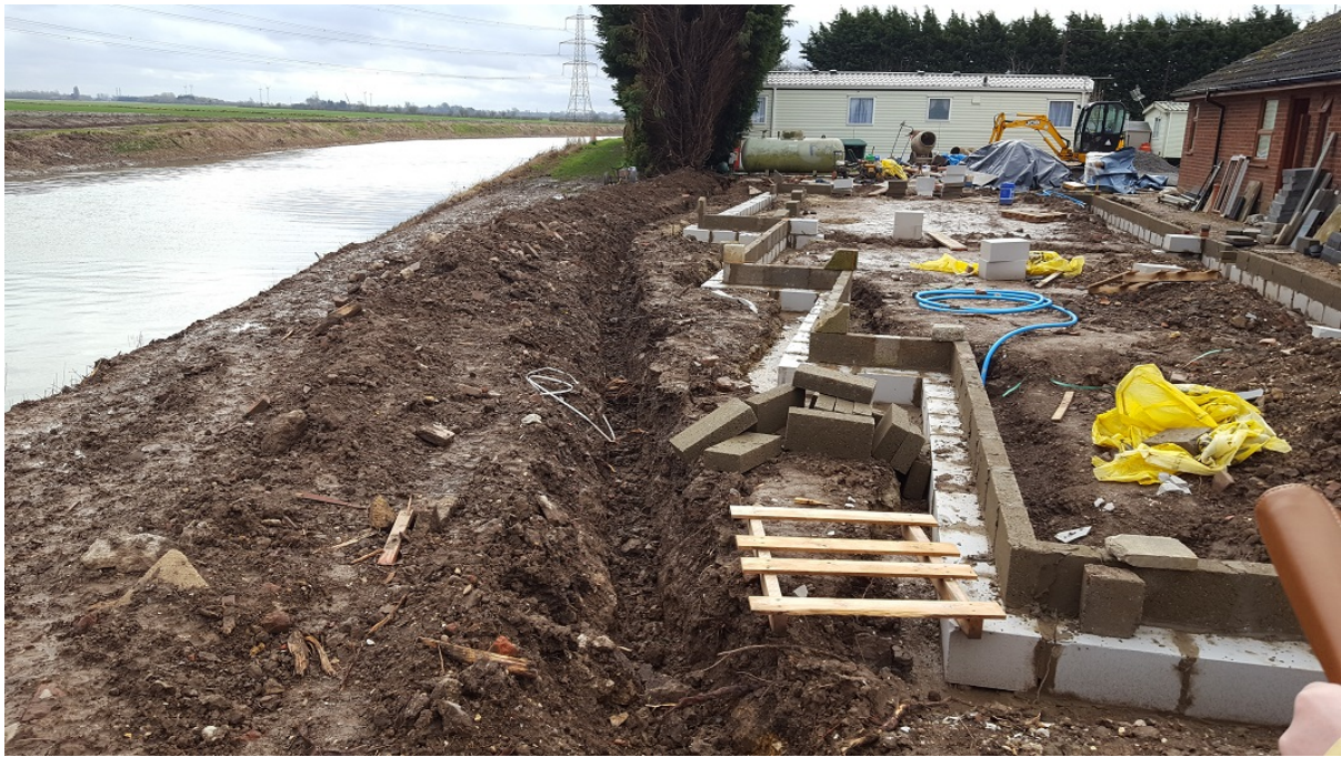
Below: Extent of current works on site
