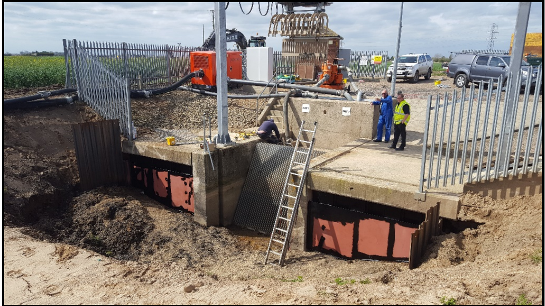
Dam across Sutton St James Drain, and over-pumping in place, to enable access to sheet piles
