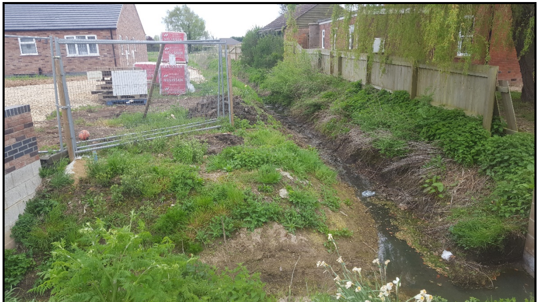
The same view following completion of the improvement works – April 2018. The watercourses are now nearly empty.
