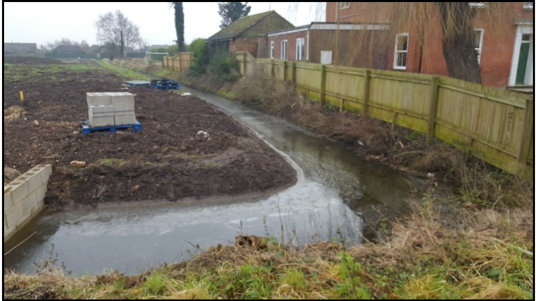
View of the private watercourses upstream of the improvement prior to works being undertaken – Feb 2017. The watercourses used to sit permanently full of water.
