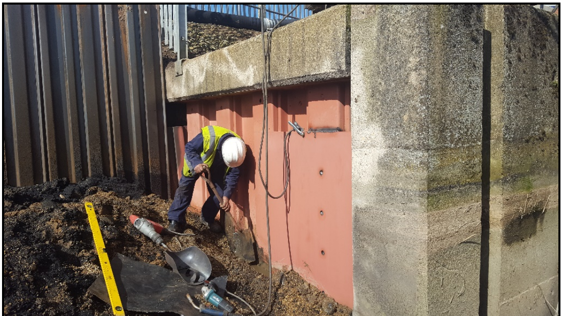
Sheet piling shot blasted and primed. New steel strengthening plates being welded in to position
