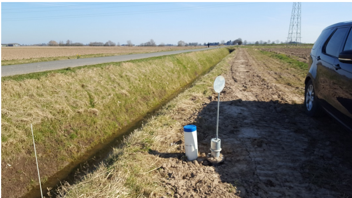
Below: Line of recently installed main with hydrant and air valve
