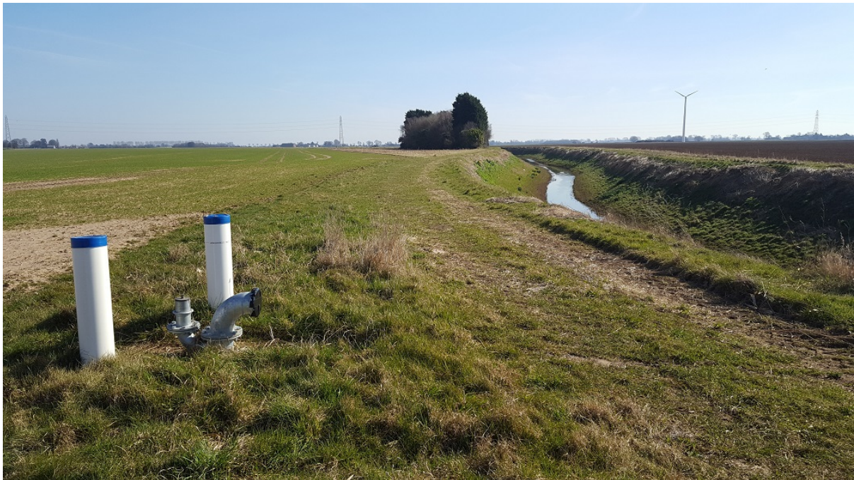
Below: Valves and connections for temporary crossing
