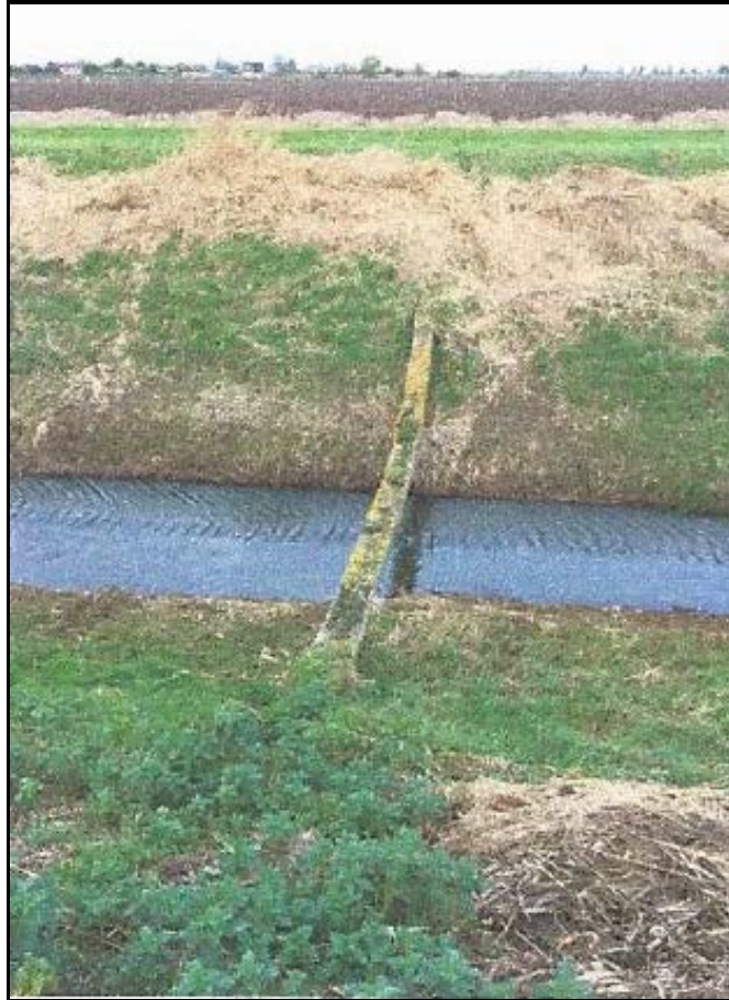
Existing wooden footbridge
