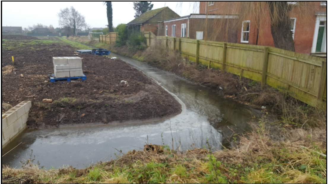
View of water ponding in open watercourses with no means of discharge
