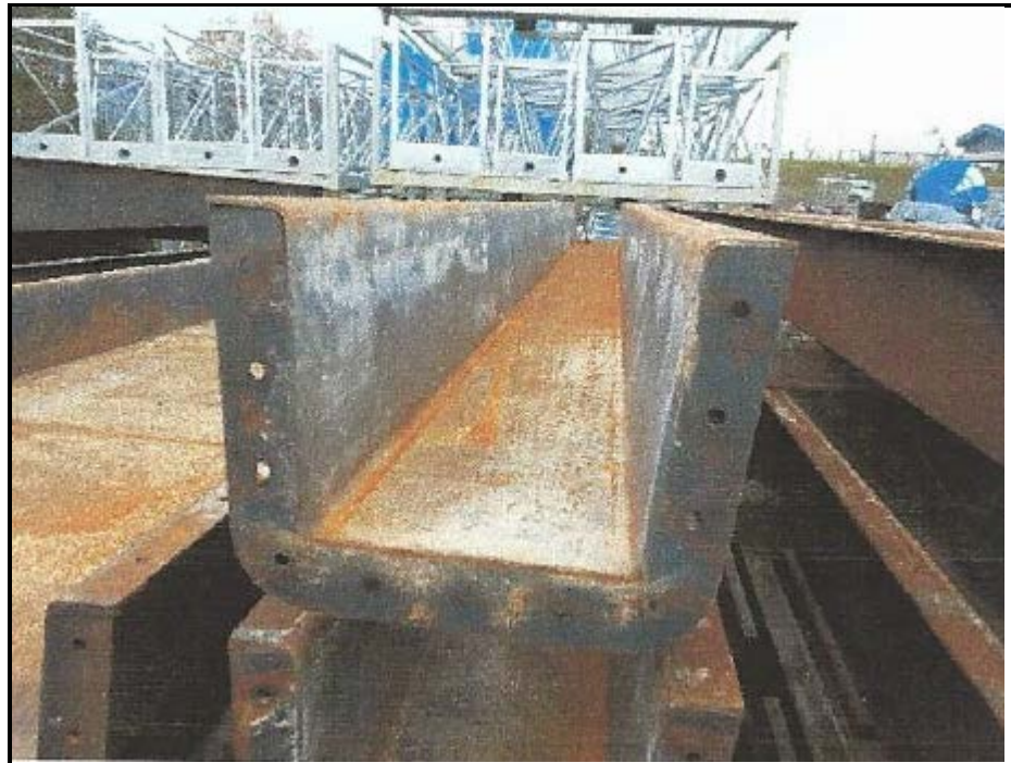
Proposed steel channel (25cm high x 28cm wide) section footbridge (200mm plastic pipe to fit inside)
