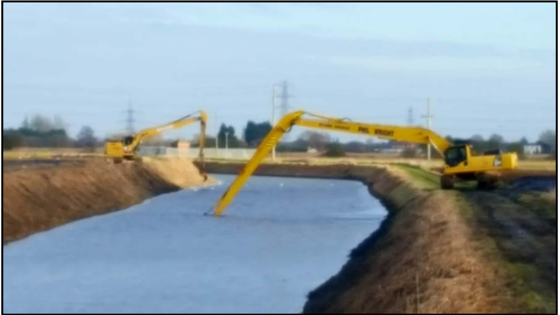
Mudding on the South Holland Main Drain
