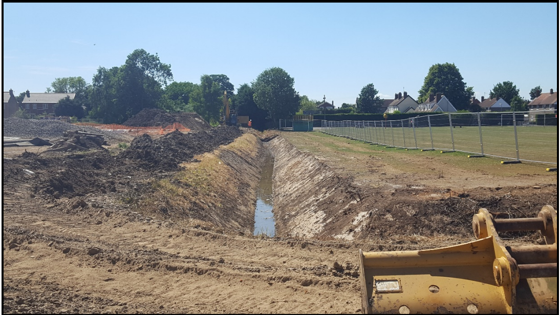
Re-profiling of Mill Dyke Branch Drain – rechargeable work carried out at the expense of the developer
