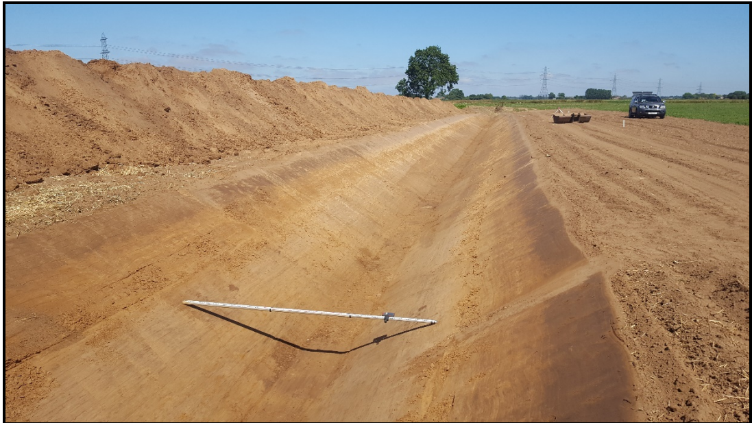
Re-alignment of Pig Lane Dyke – section of new cut
