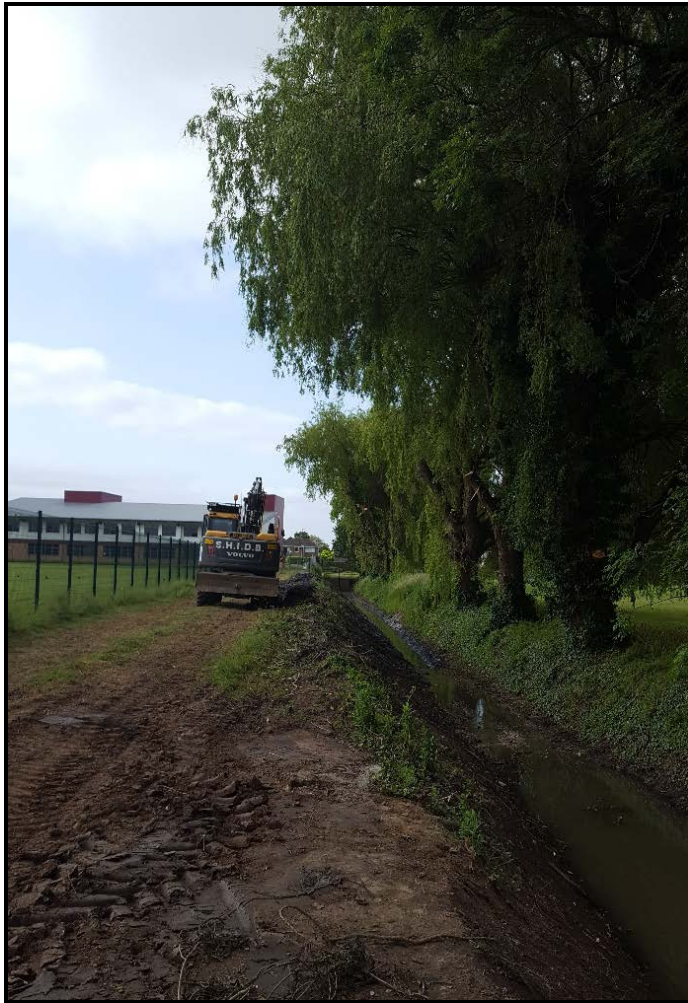
Willow trees after pruning, allowing machine access to drain
