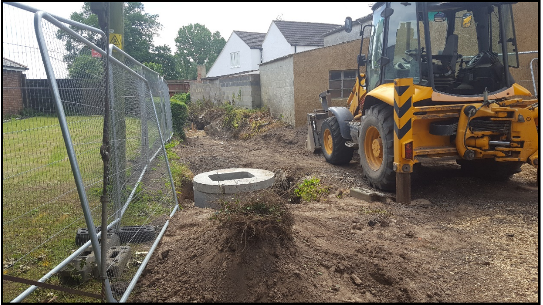
Piping of upstream section of Scarlet Gate Drain, work in progress, June 2018.
