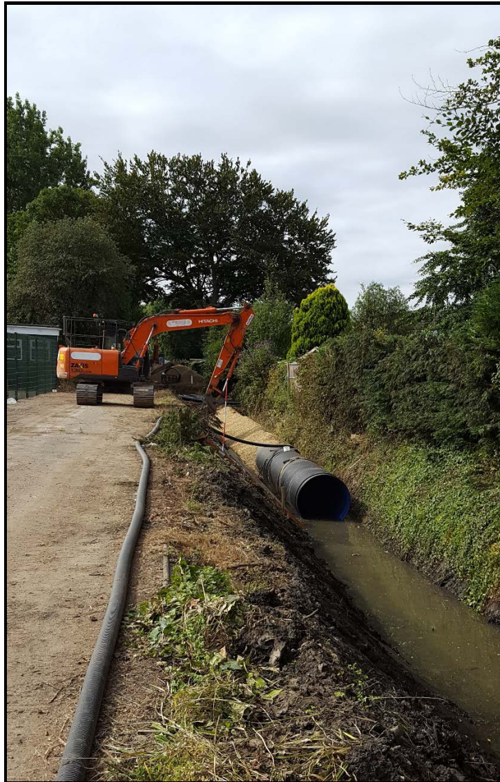
1.2m dia plastic pipe being installed – July 2018
