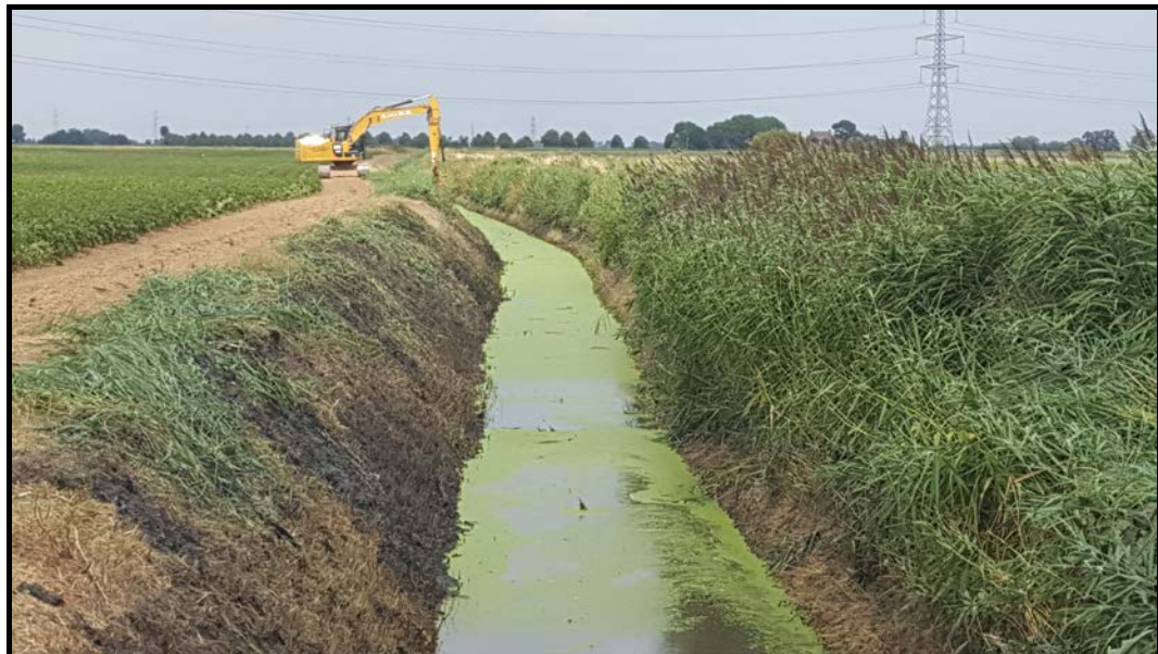
Board's excavator basket cutting Lords Drain – July 2018
