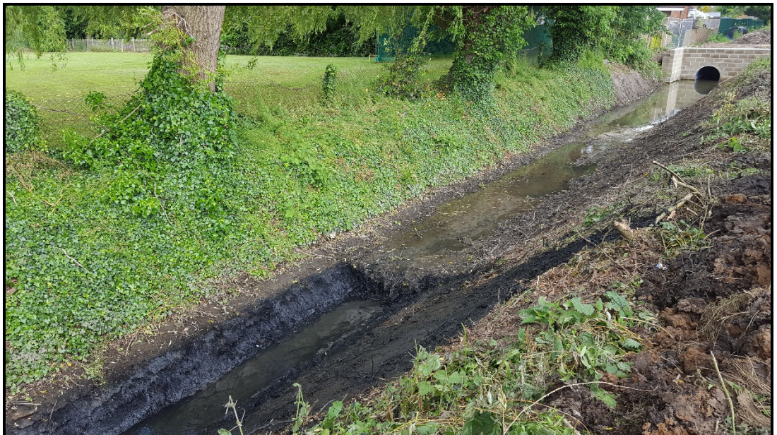
Years of mud and debris build up being removed from bed following machine access being made available
