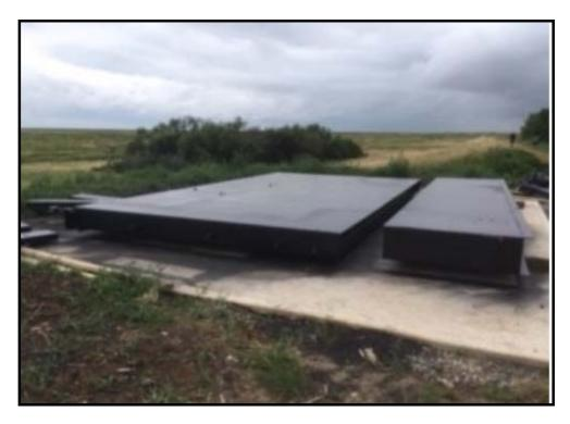
Sluice Door and Counter Balance shot blasted and painted ready for installation
