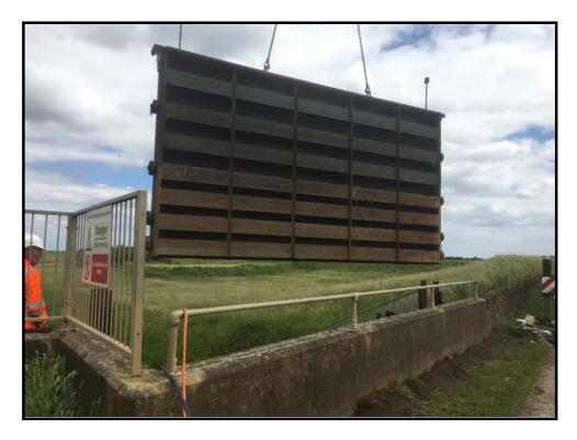
Removing the sluice doors with 60t Crane
