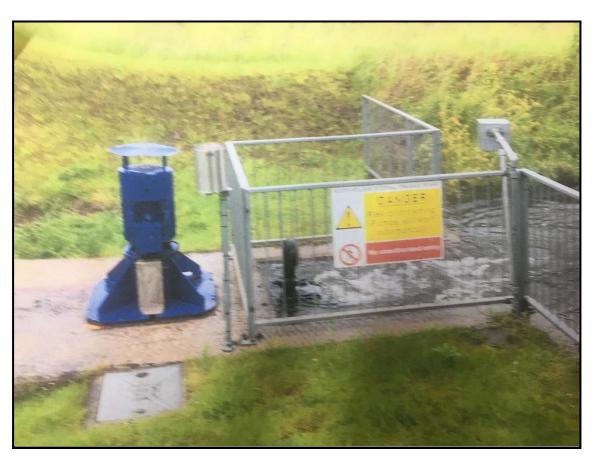
Manor Farm Pumping Station outfall, 13 June 2019. Downstream water level threatening to flood pump.
