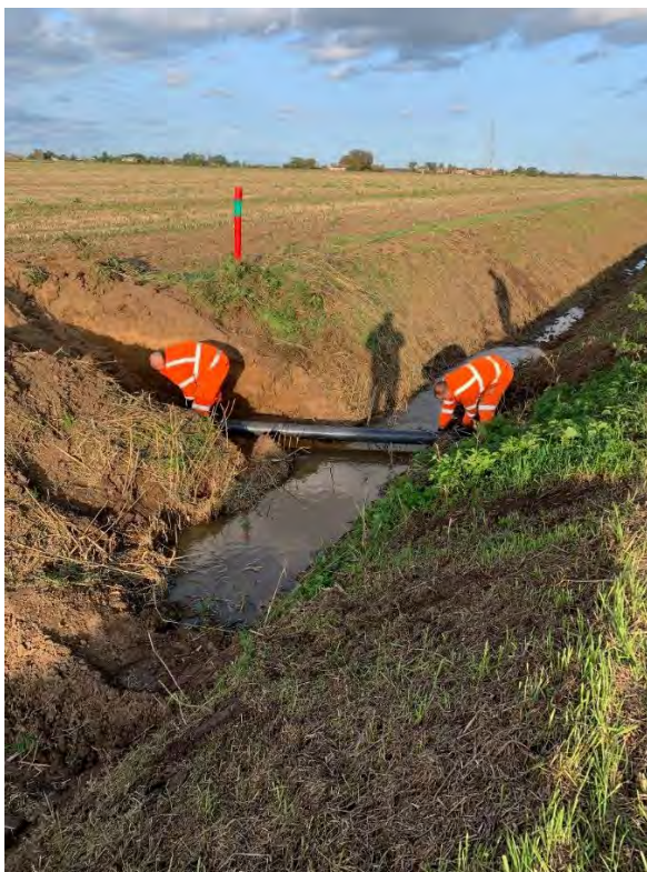
View showing earth bund in position to contain leakage (left) and Anglian Water undertaking repair (right)
