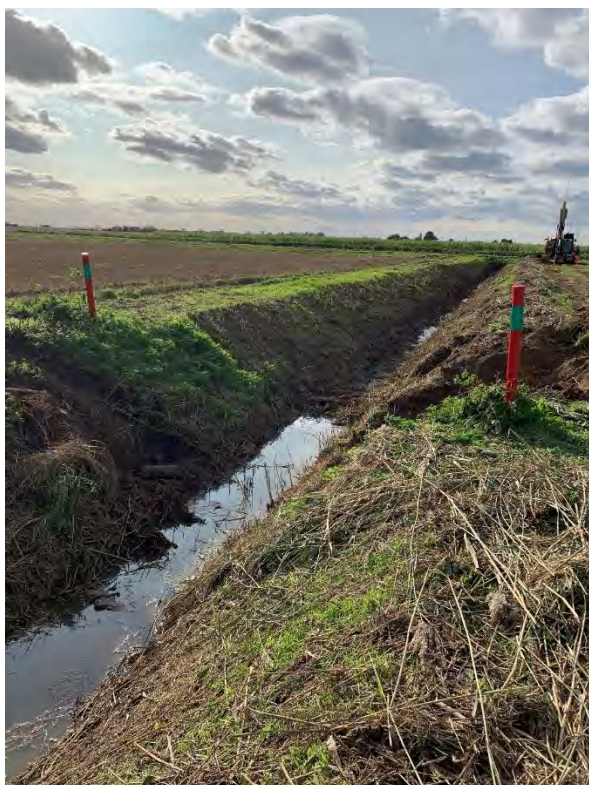
View showing earth bund in position to contain leakage (left) and Anglian Water undertaking repair (right)
