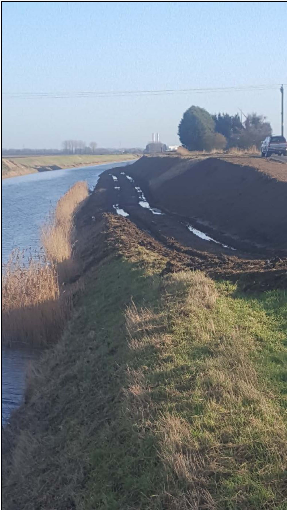
Berm reinstatement between Sharpes Bridge and Wisbech Road
