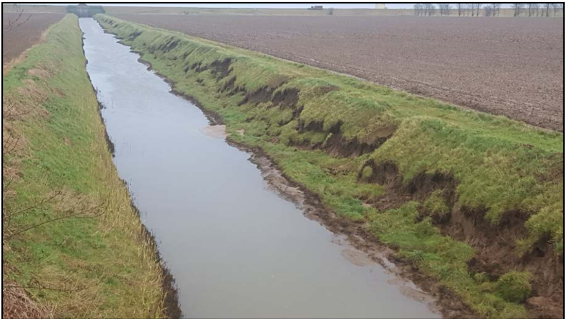
Bank slips along Dawsmere Drain from second line sluice to pumping station
