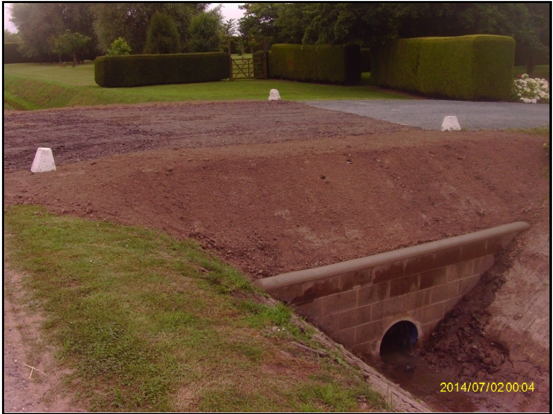
New culverted access built in 2014
