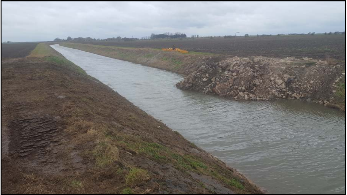
Railway bridge removed
