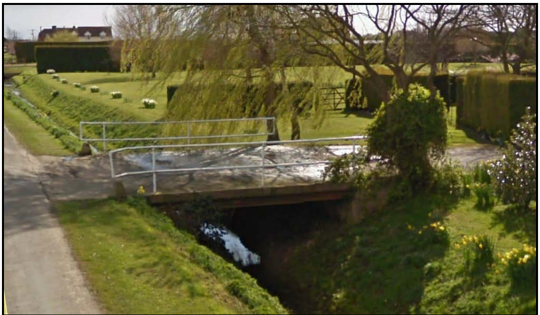
Original free span bridge access
