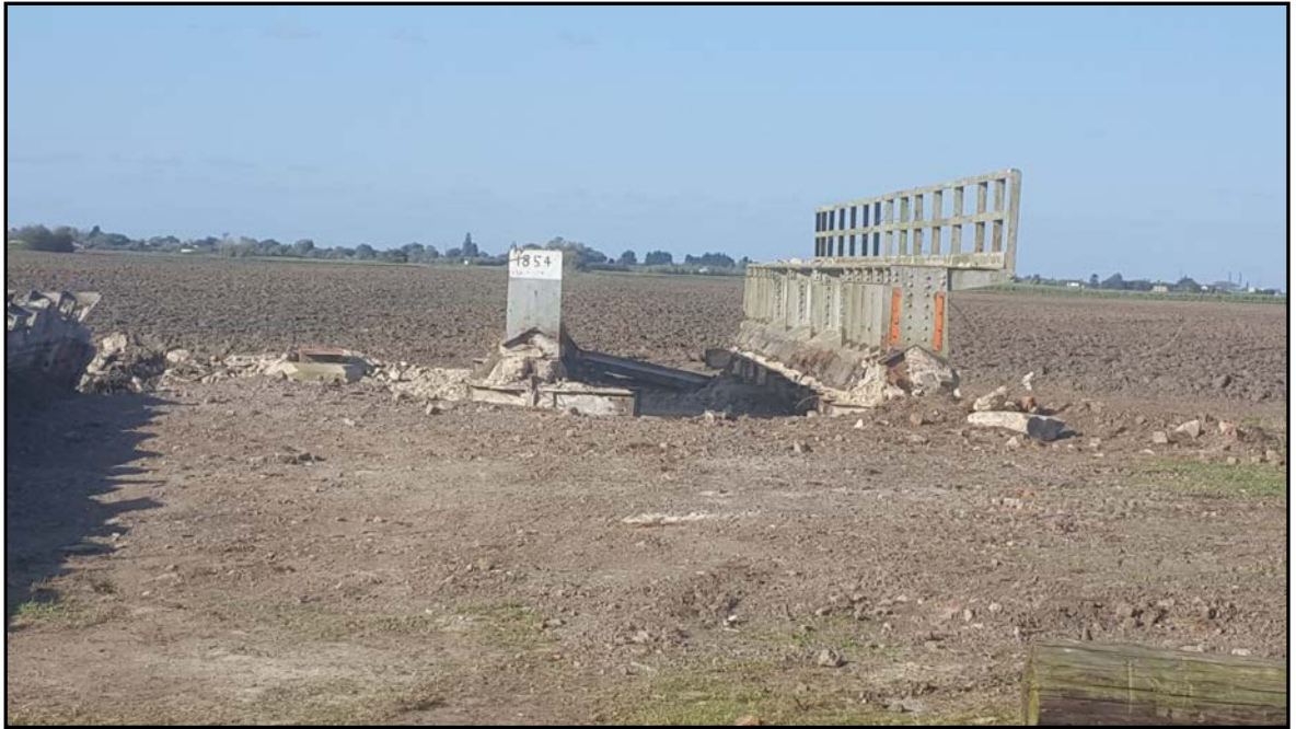
Removal of old railway bridge
