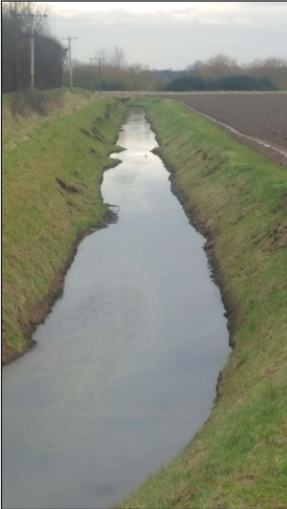
Bank slips along Dawsmere Drain from second line sluice to duck pit
