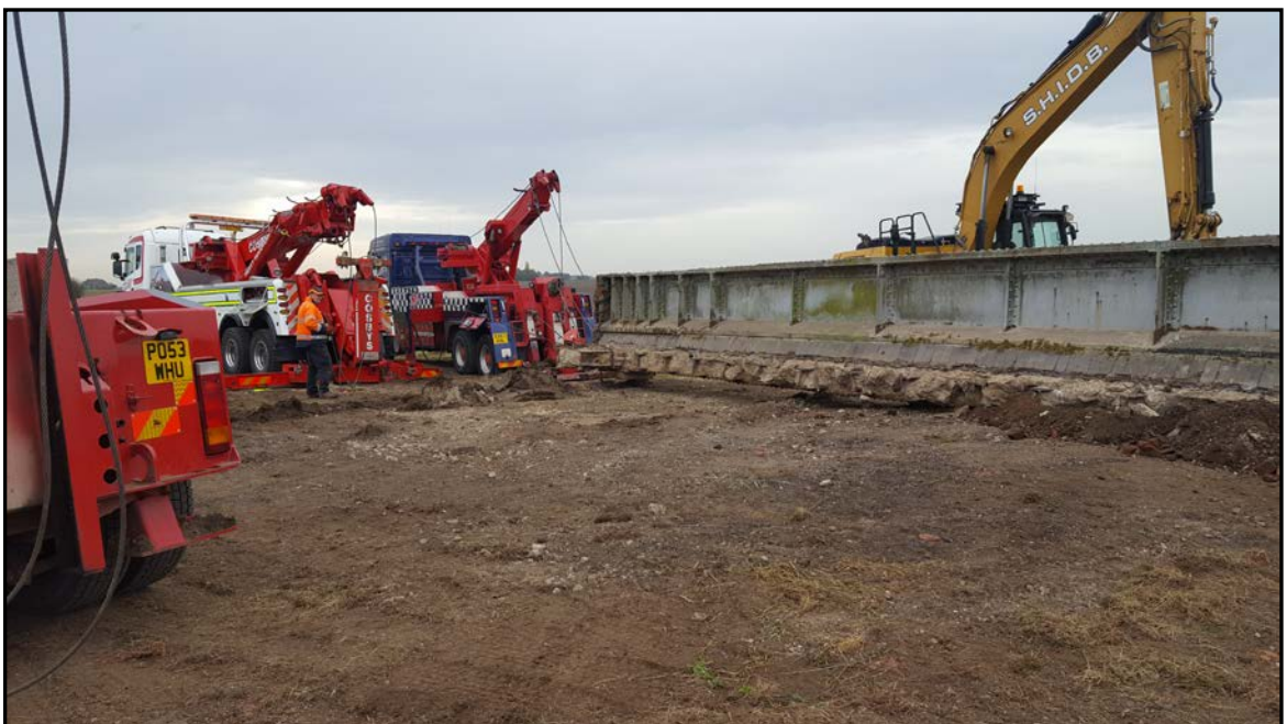
Removal of old railway bridge
