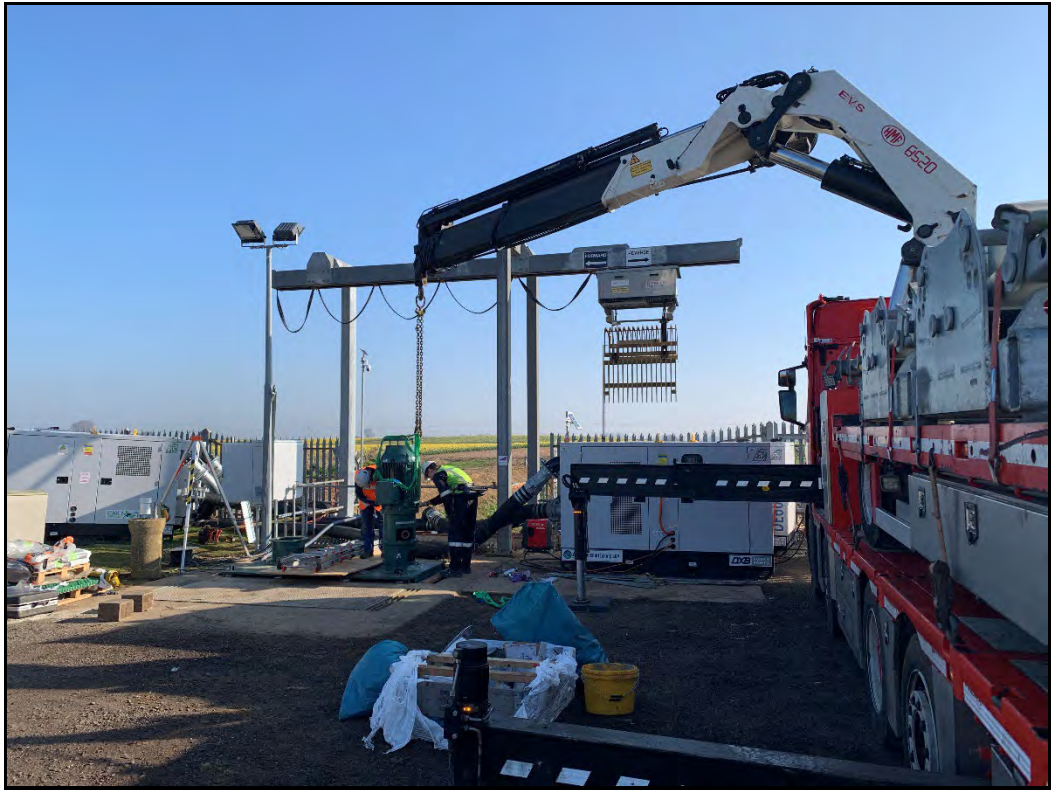
Lifting one of the new motors into position
