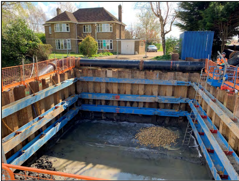
Excavation dug to foundation level
