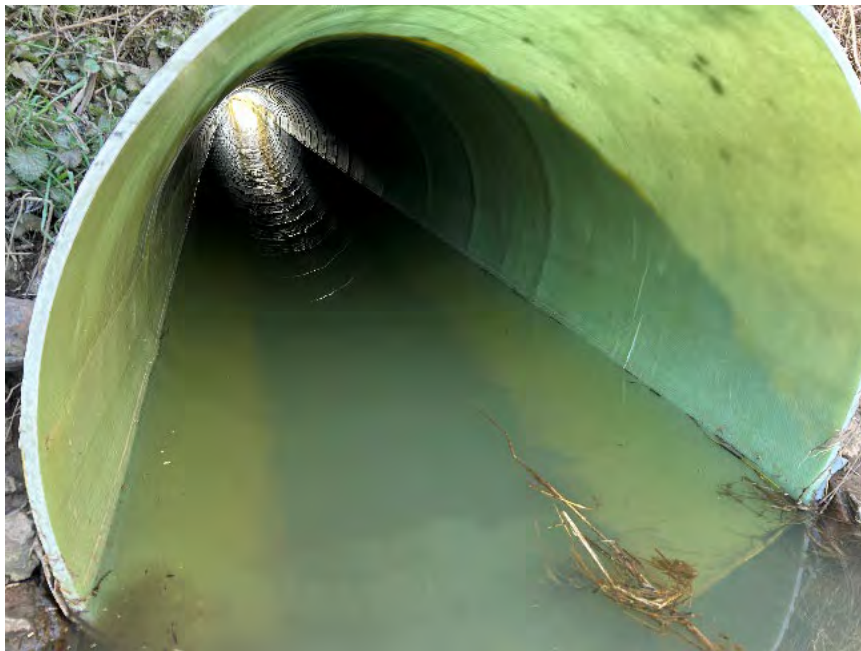
View of one of the lined culverts, and an example of a recently completed headwall
