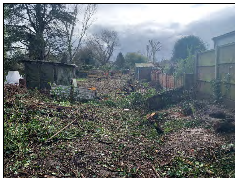
Views along route of Pipeline 1 immediately following tree/vegetation clearance – Feb 2026
