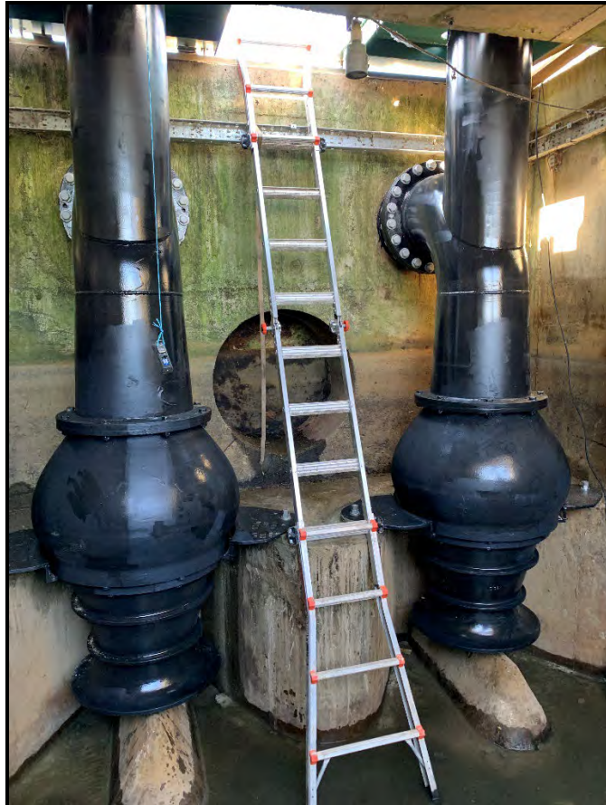
Pumping station sump dammed off and pumped out - new pumps installed
