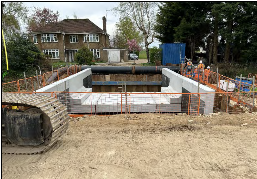
Precast box sections and headwalls installed
