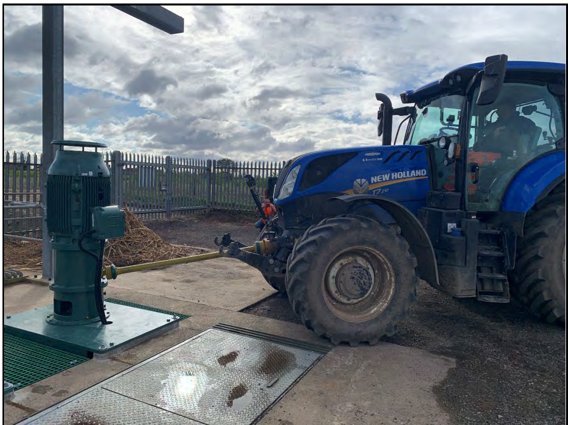
Testing PTO drive on pump
