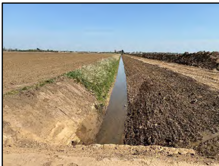
Reprofiling works on Bulb Company Drain, Low Fulney.
