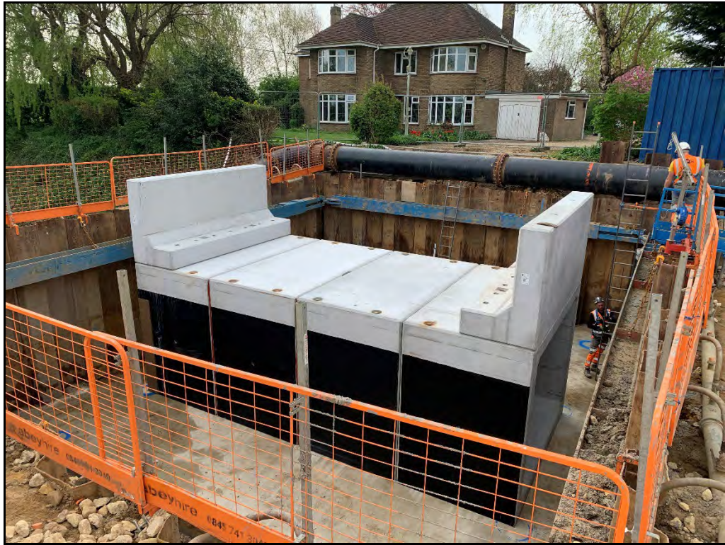
Precast box culvert sections in place
