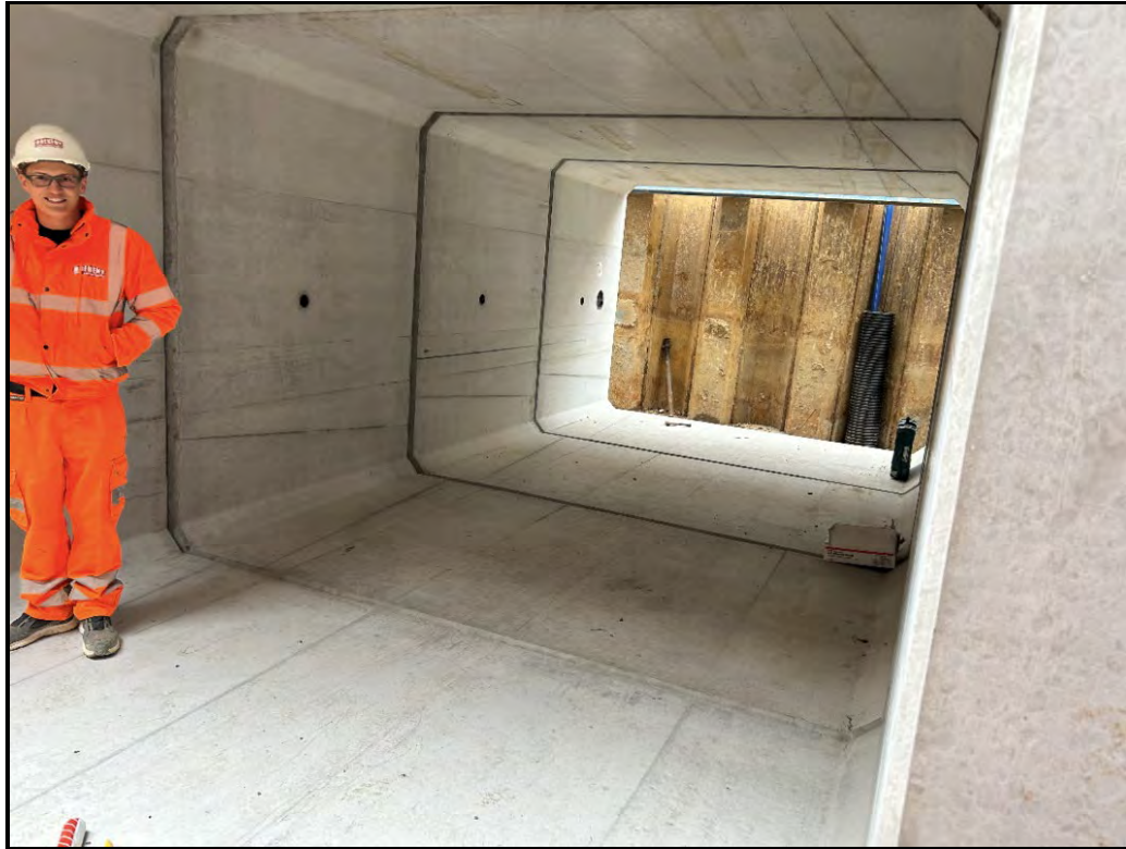
Inside precast concrete box sections
