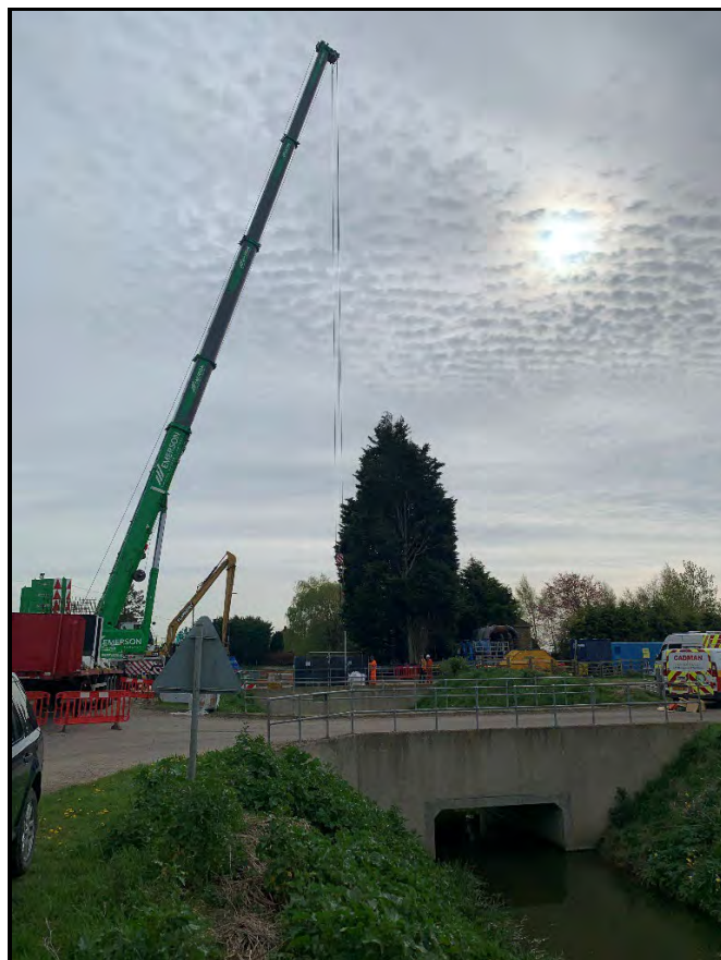
400 tonne crane lifting in the precast concrete units
