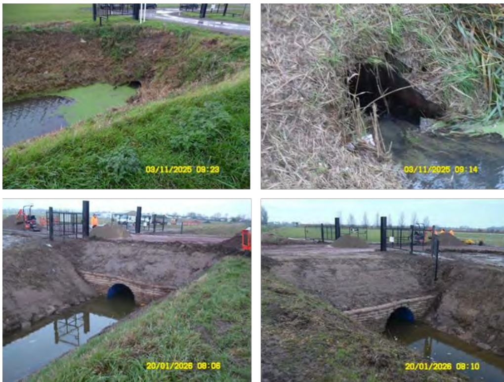
Figure 2: Photographs of the culvert before (top) and after (bottom) works.
