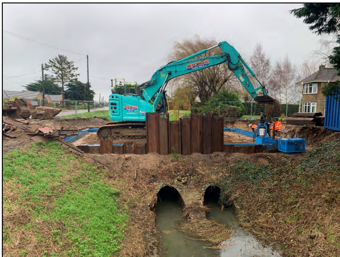
Cofferdam in the process of being installed – Dec 2025
