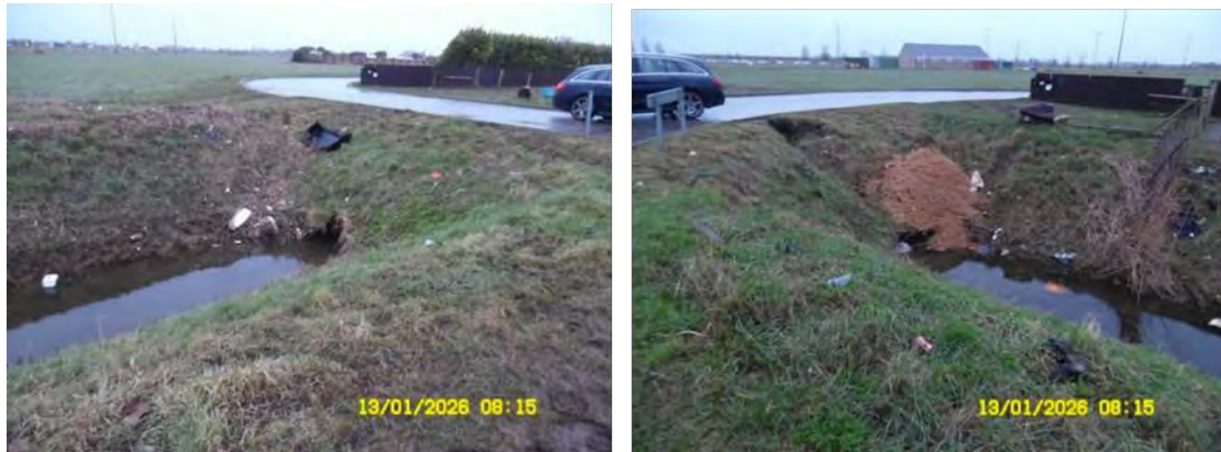
Figure 3: Photographs of the culvert carrying Evergreen Close.
