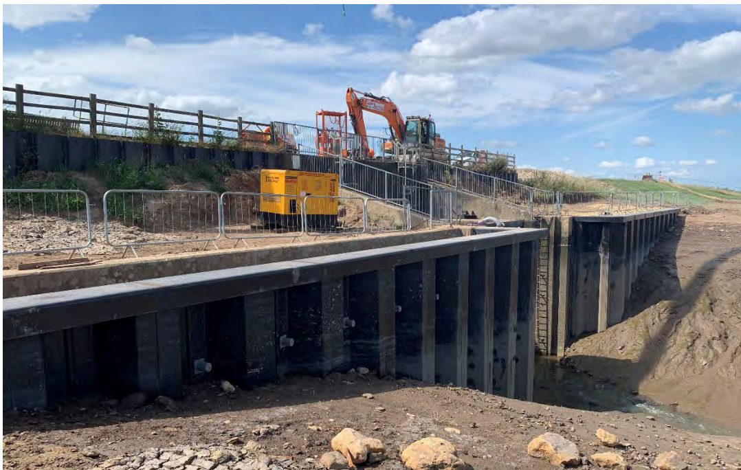
View of new tidal sheet piling wing walls and capping beams
