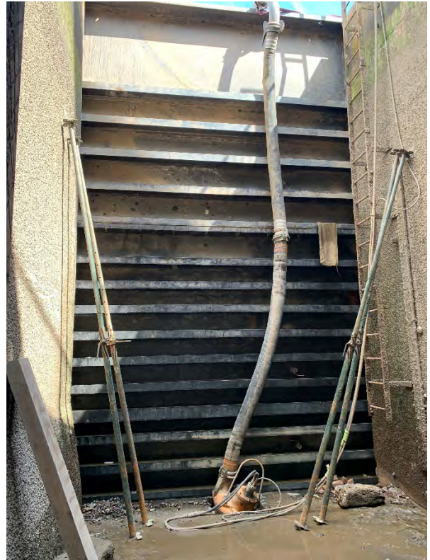
Tidal dam door in position View from above (left), internal view showing box culvert de-watered (right)
