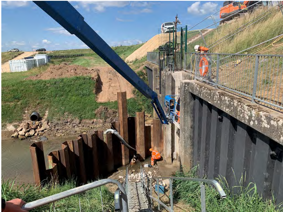
Upstream view showing freshwater steel pile dam, and operations to remove old freshwater door frame
