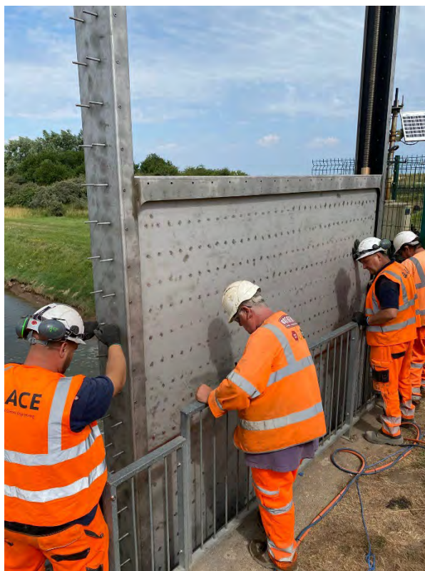
Installation of new freshwater penstock on southern box culvert
