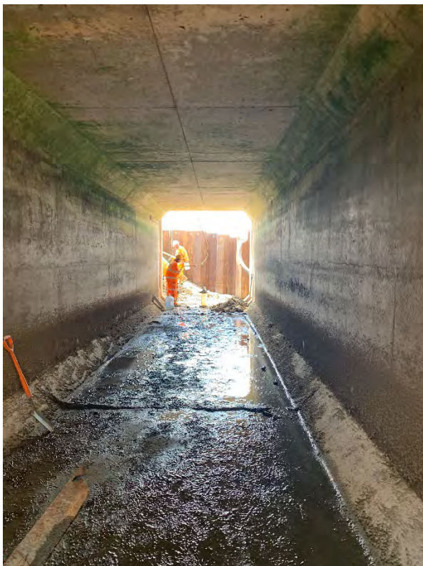
View of southern box culvert de-watered and cleaned out (left), and removal of old tidal door frame (right)
