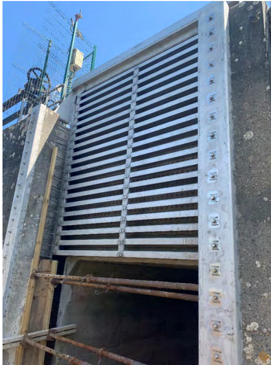
New freshwater penstock anchored into position
