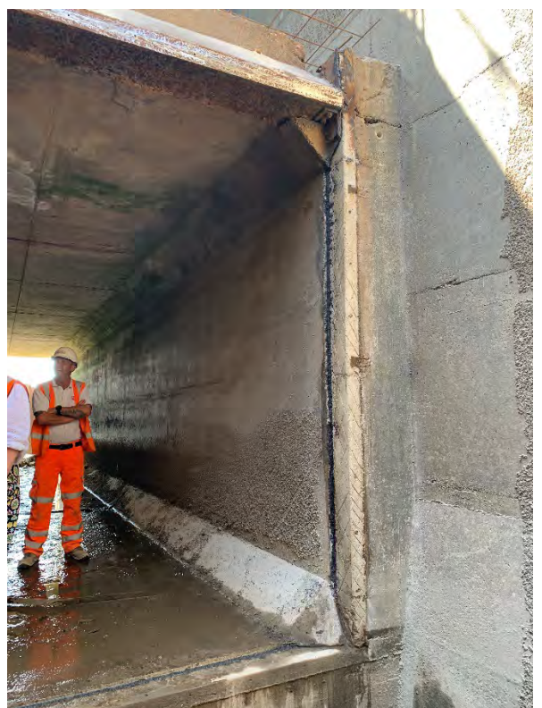
View of southern box culvert de-watered and cleaned out (left), and removal of old tidal door frame (right)
