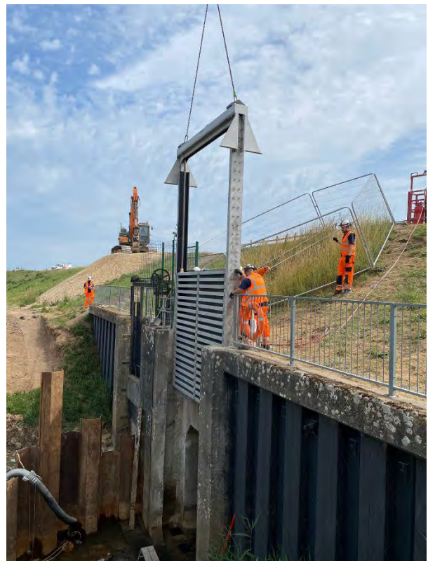
Installation of new freshwater penstock on southern box culvert
