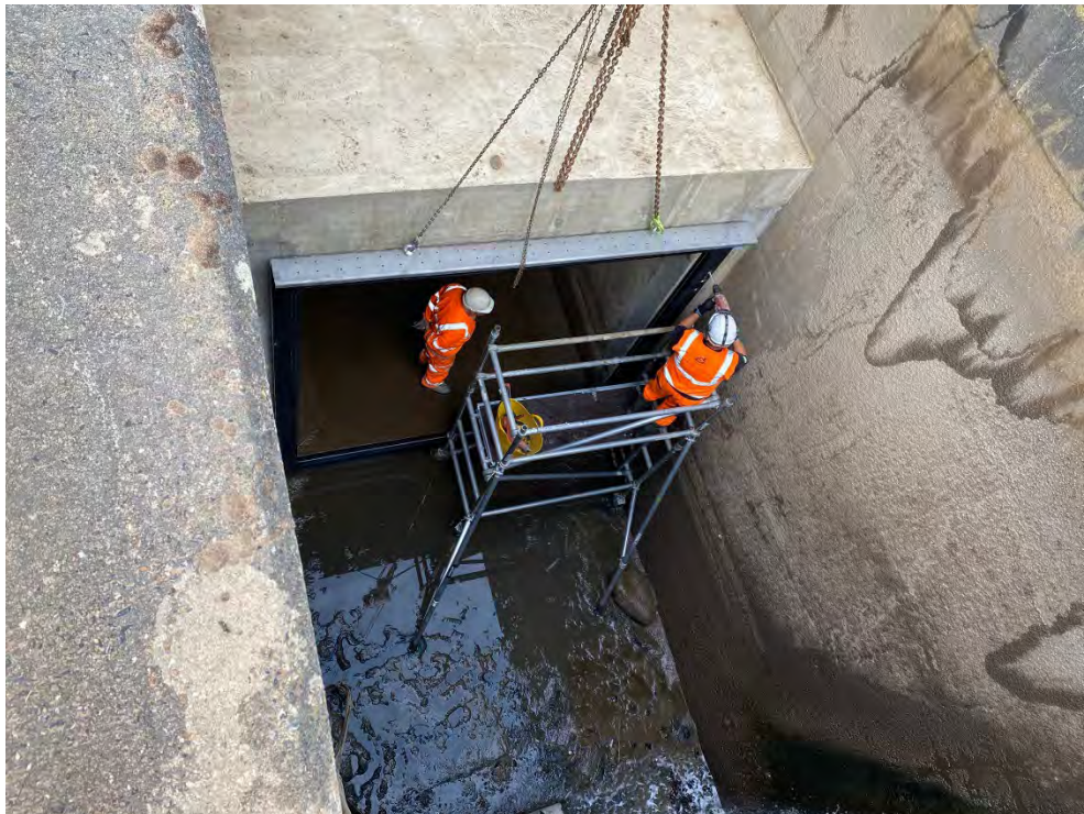
New tidal flap frame being installed
