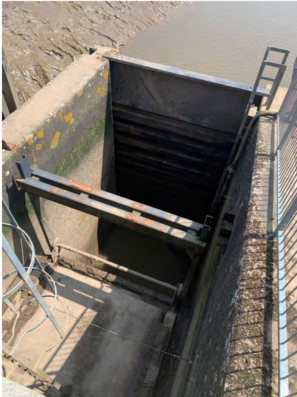
Tidal dam door in position View from above (left), internal view showing box culvert de-watered (right)
