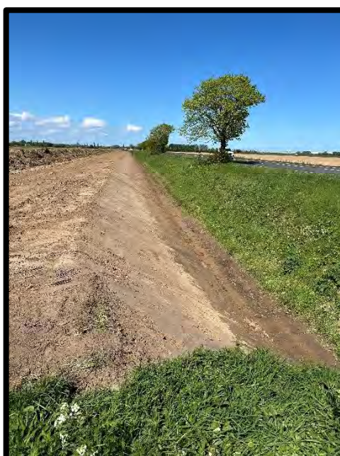
Reprofiling works on Wisbech Road Drain, Long Sutton.
