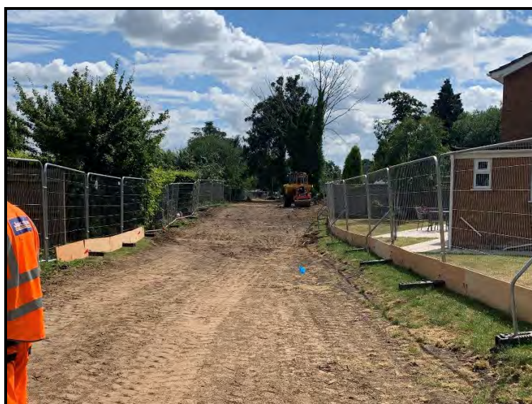
Views showing establishment of working corridor along route of Pipeline 1 – Jun 2026
