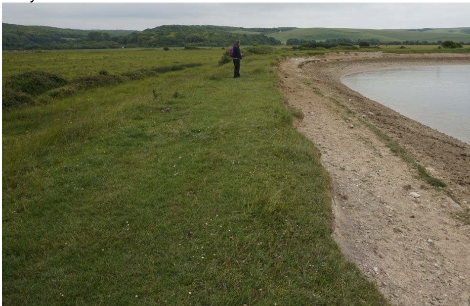
Example of bank cliffing, which will ultimately erode the bank.
