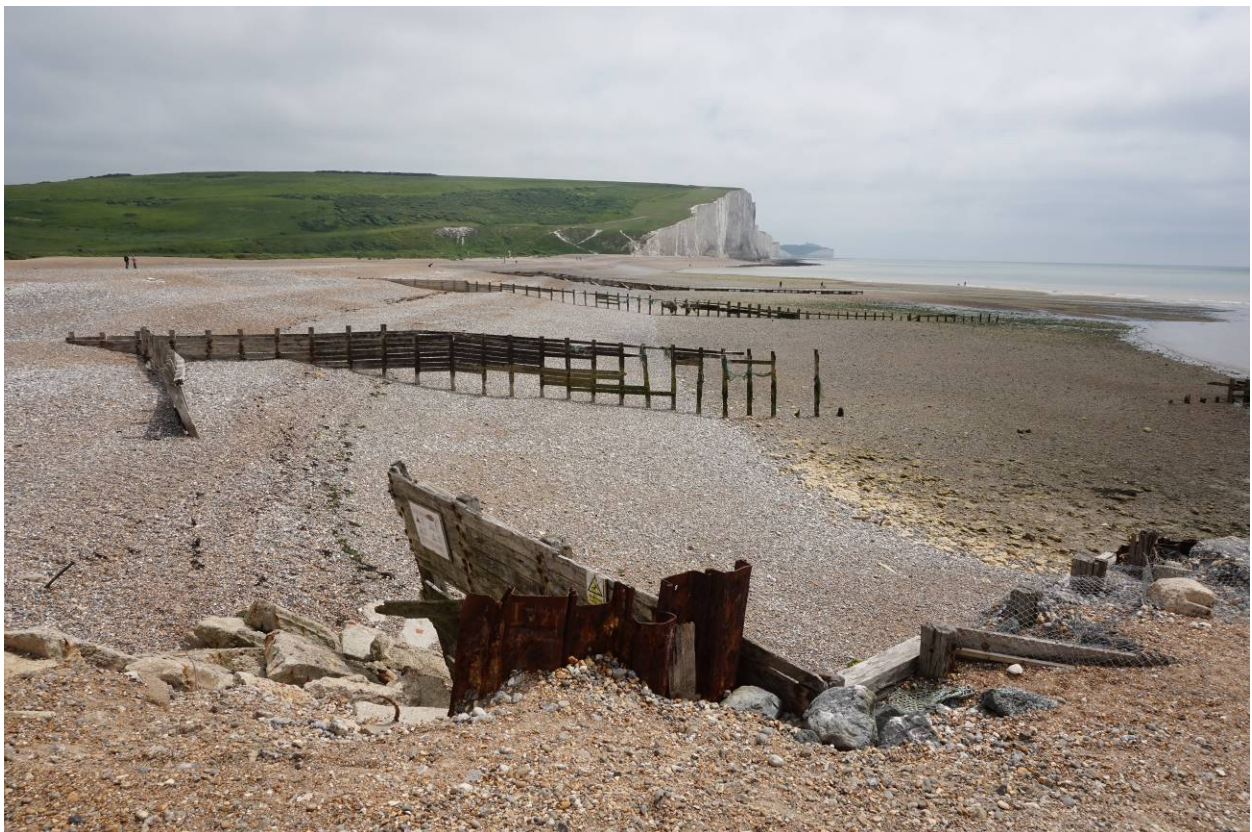
Heavily degraded groynes at river mouth, which could be refurbished
