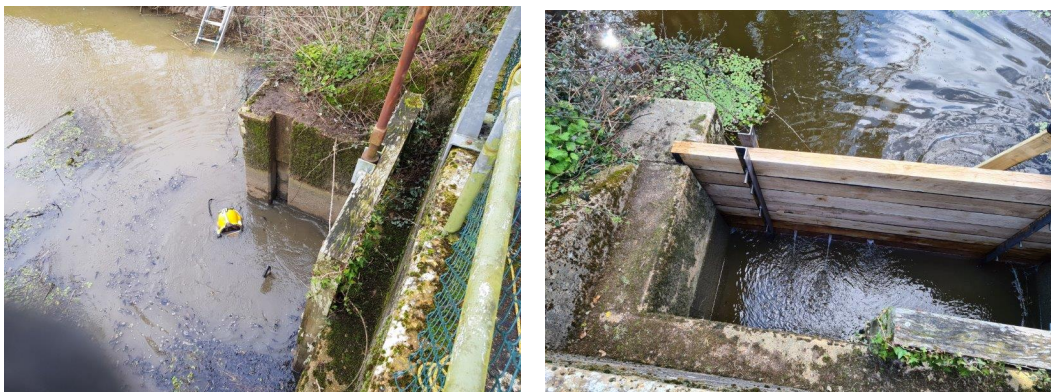
Diver clearing debris from the channels within which the sop log sits and the stop log installed
