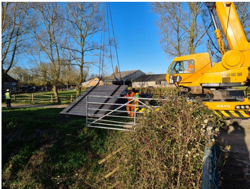
New stop log being lifted into position
