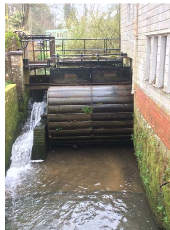
Hellingly Water Mill – Mill laid
