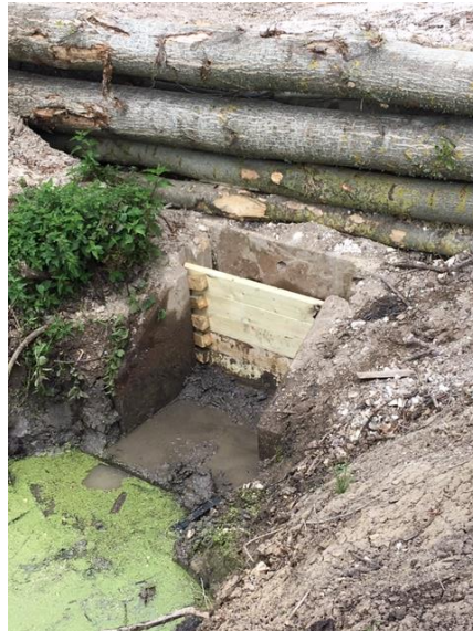
New Dam Boards at two sites on the Marland
