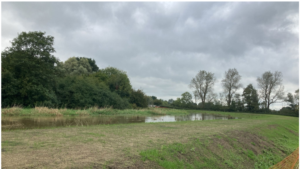
Figure 3: Embankment in November 2024
