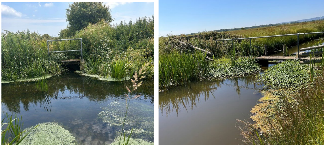
Figure 8: Water Control Structures at White Dyke and Rickney Sewer in June 2024
