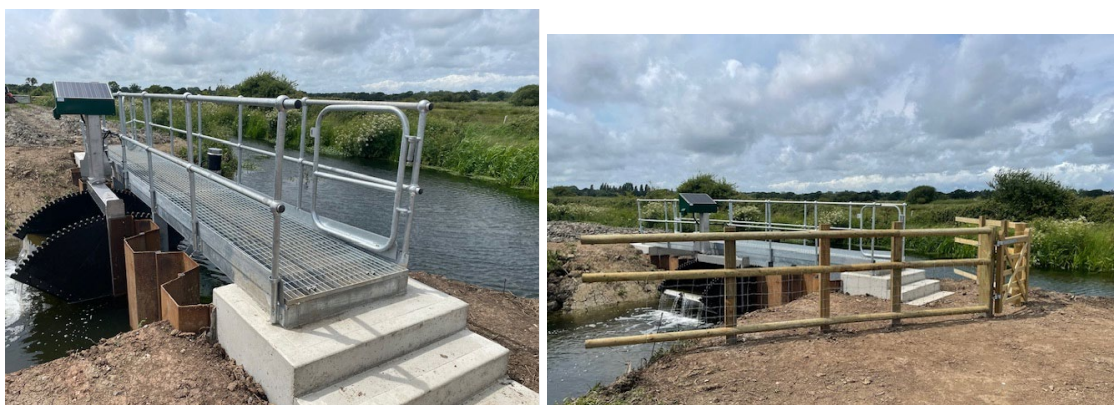
Figure 9: Tilting Weir Installed on White Dyke Sewer
