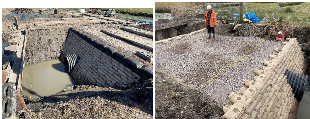
Figure 7: Horse Eye Culvert During Construction in March 2025
