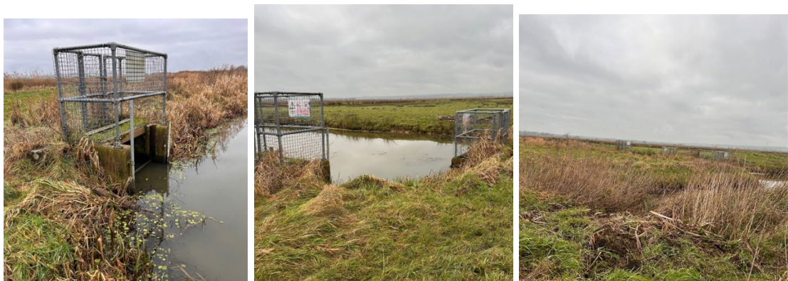
Figure 12: Photos of existing structures at Spaghetti Junction
