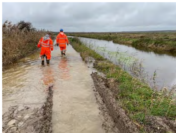
Figure 1: Flooding of Site Access
