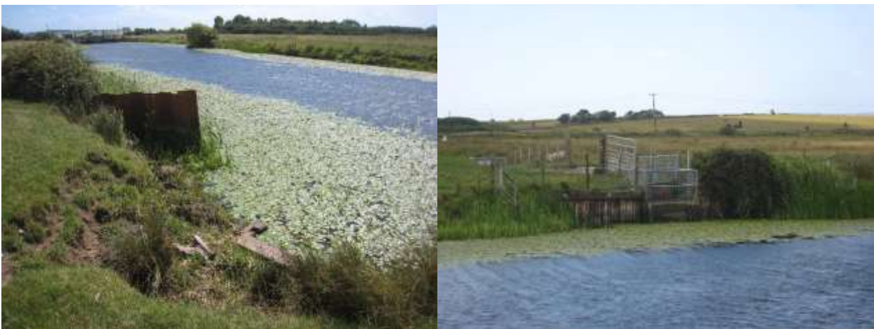
Figure 2-2 Feed structure S35 (left) and P37 (right) along the Wallers Haven high level carrier
