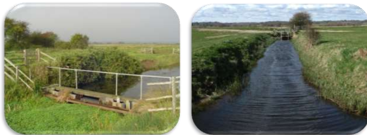
Figure 2-3 Retaining structures R42 and W42 in the Horse-eye drainage area along pumped drained ditches
