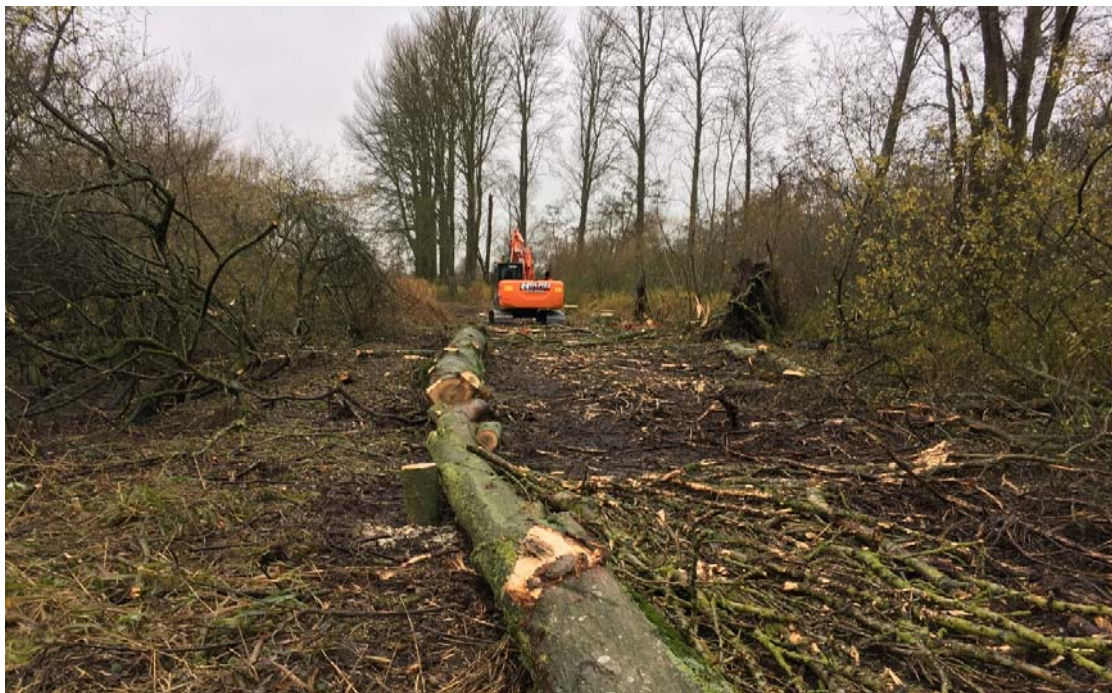
Leaky dams installed from locally felled Poplar trees
