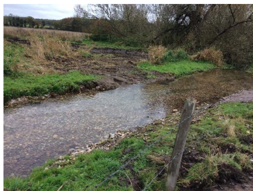
Bed raising using gravels
