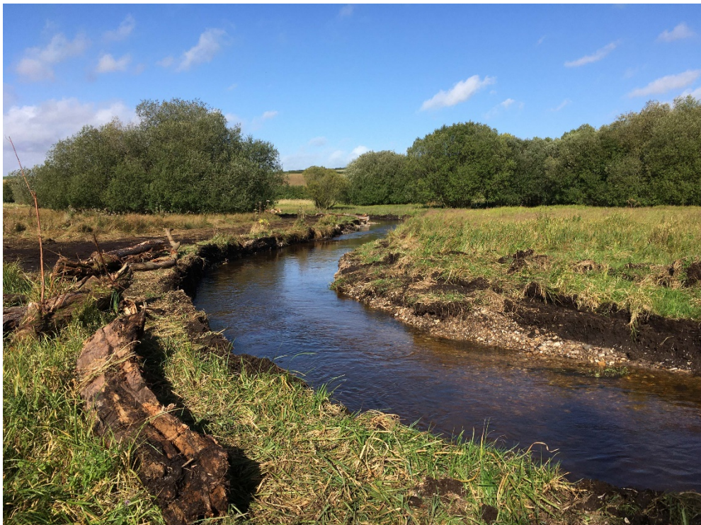
Channel completed with logs ready to be placed in the channel as woody debris.
