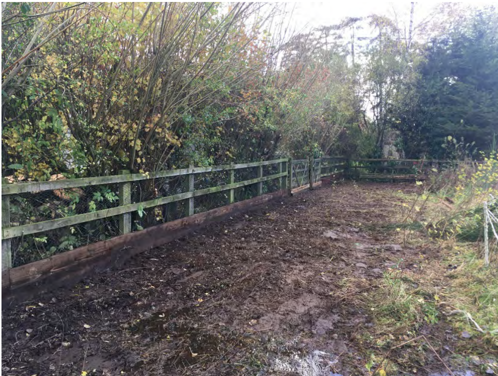
The above photograph shows how timber gravel boards have been retrofitted to existing fencing, to retain and store flood water in a paddock upstream of the properties at risk.
