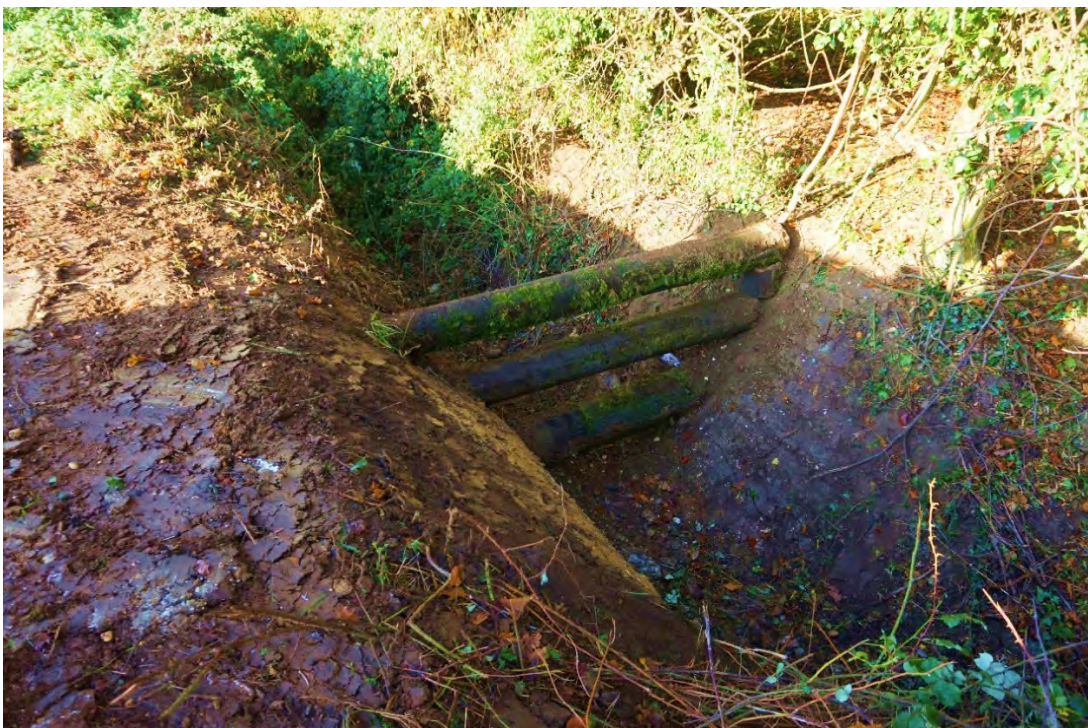
As built installation of dam with space for water to pass through.
