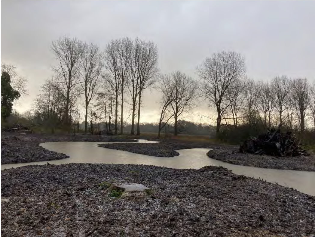
As built photograph of new channel
