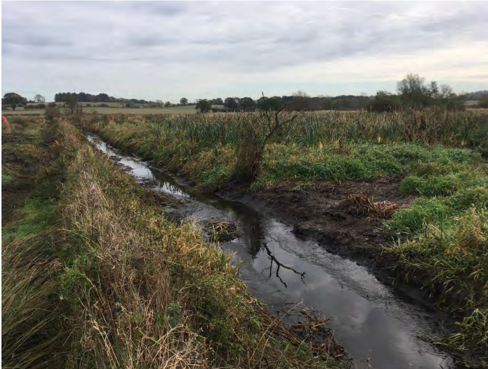
After works at Great Ryburgh B
