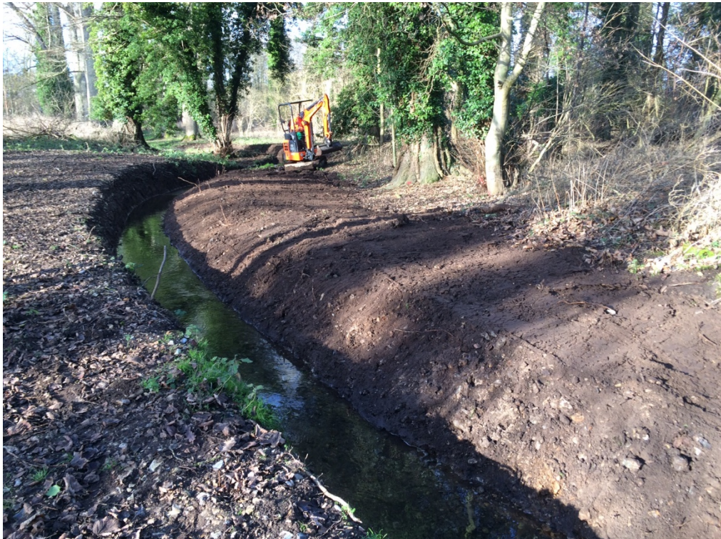
As built photograph of the modified bypass channel
