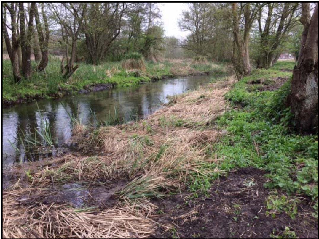
Bank and bed regrading
