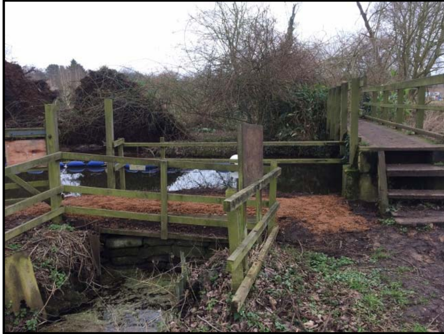
Completed bank repair at Hautbois
