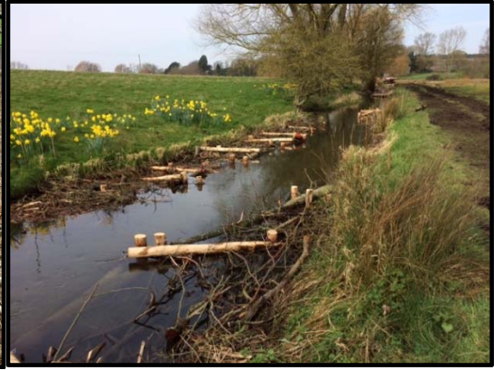
In-channel Wood Berm
