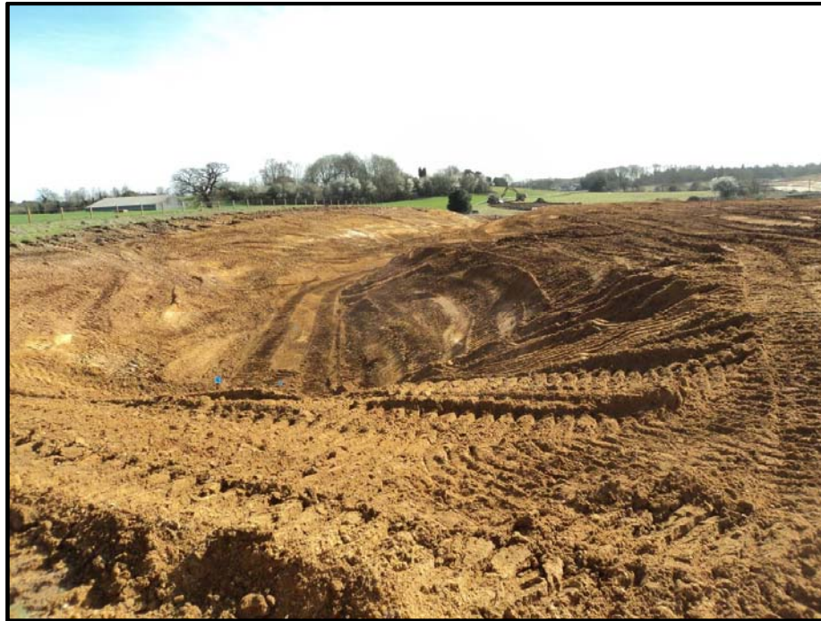
Settlement pond in construction – March 2017
