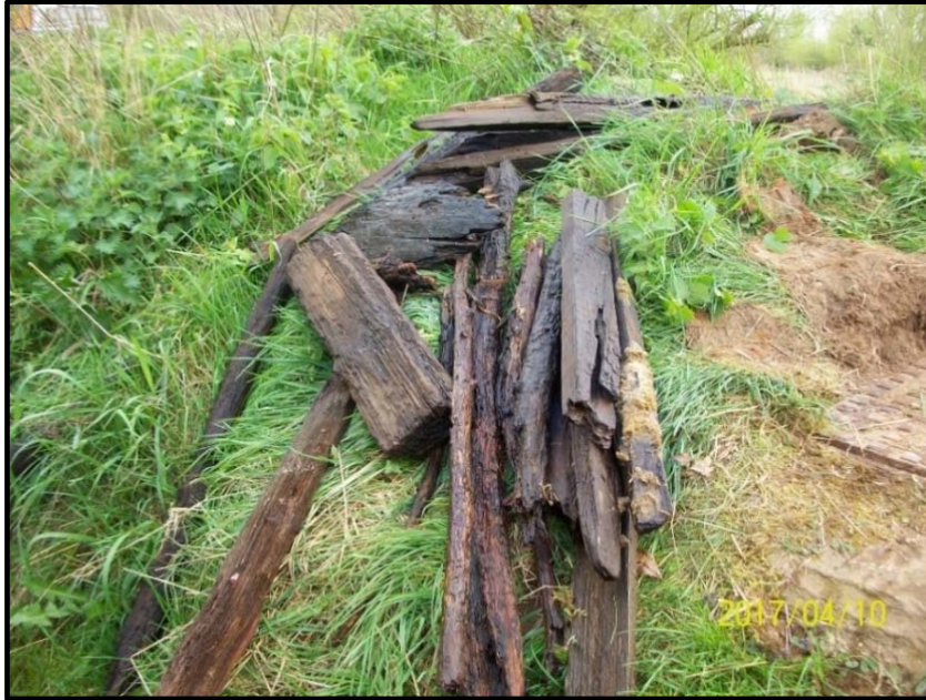
Timber debris removed from the culvert
