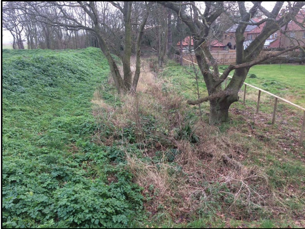
Current drain condition
