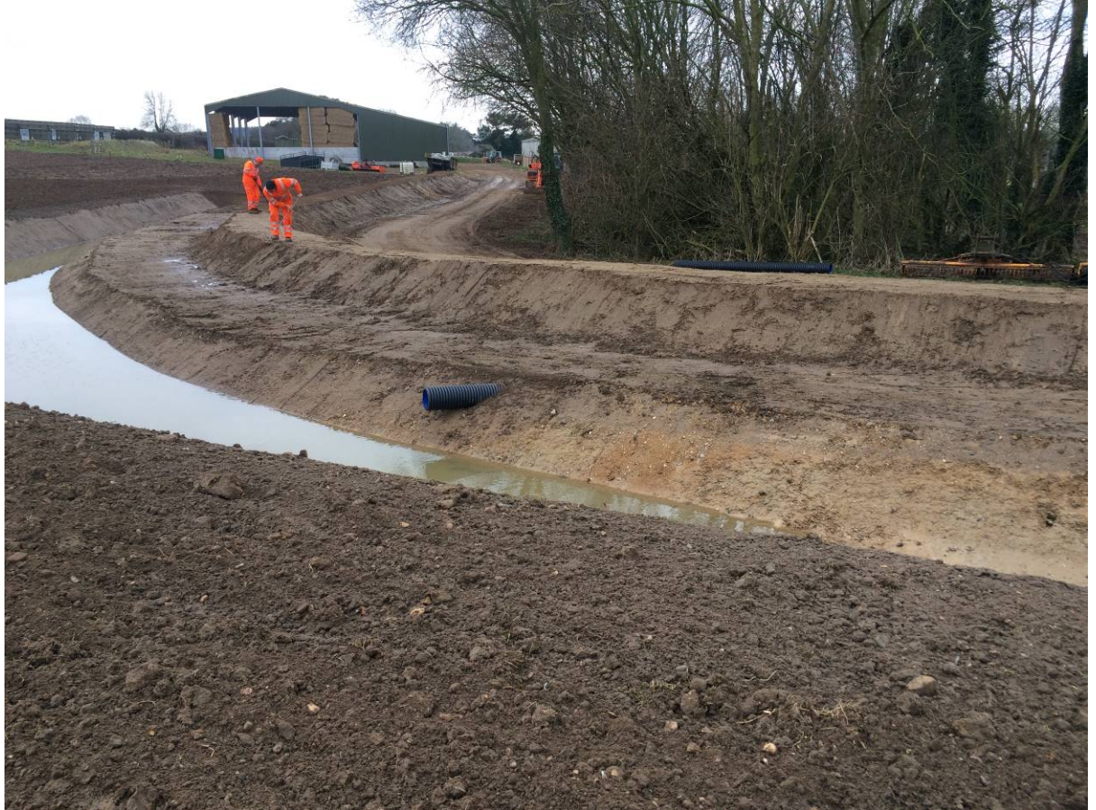
Swannington Silt Trap
