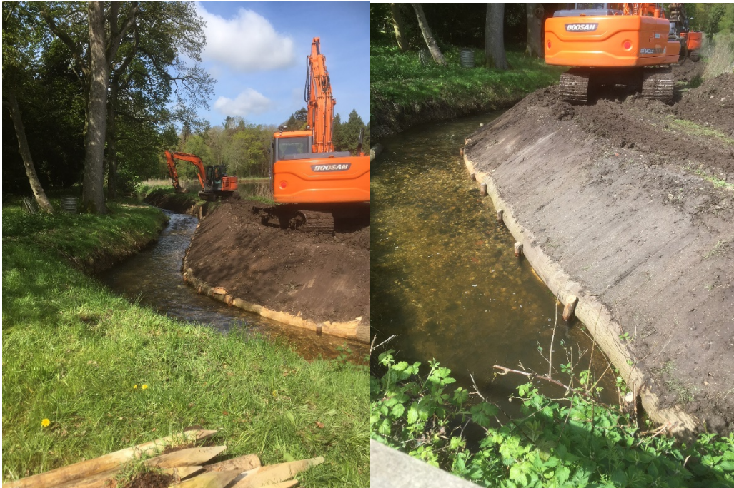
New re-profiled bank with toe protection
