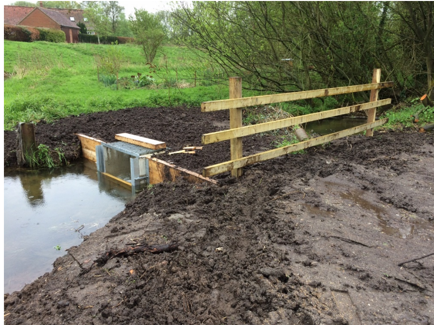
New precast structure
