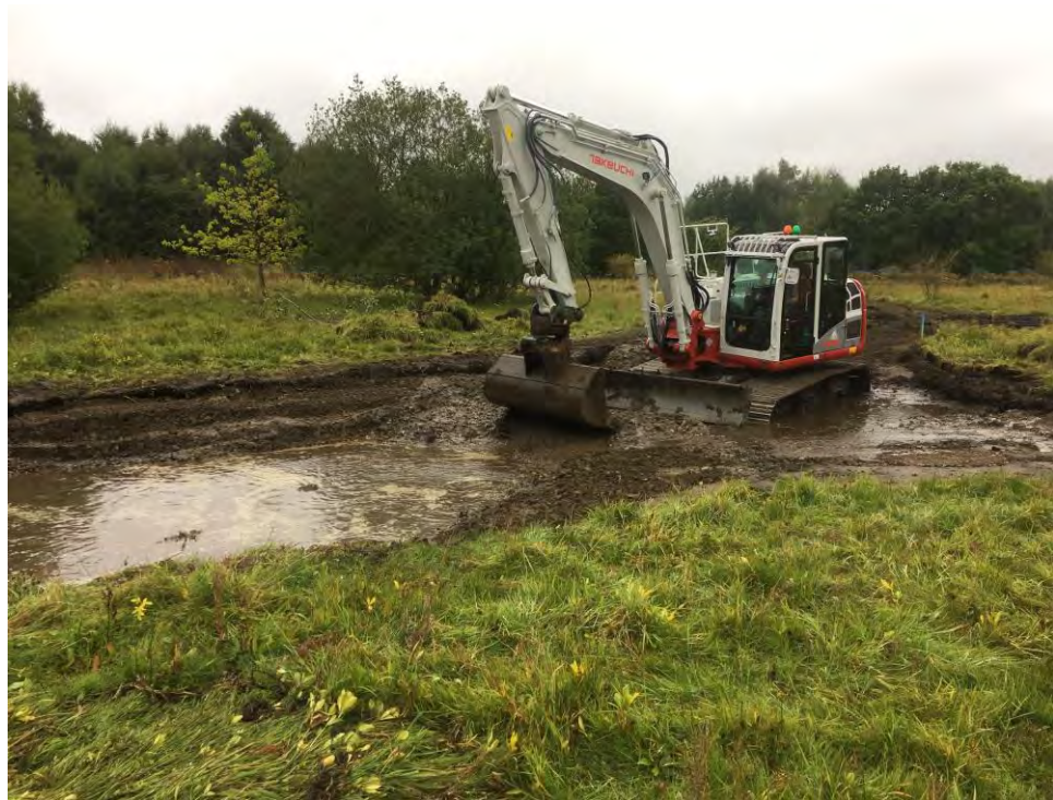
Excavator with wide tracks constructing the new channel
