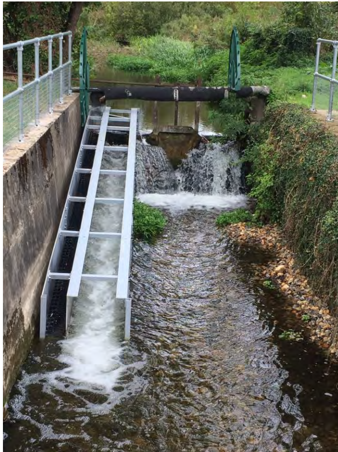
Fish and Eel pass in place (IDB Drain)
