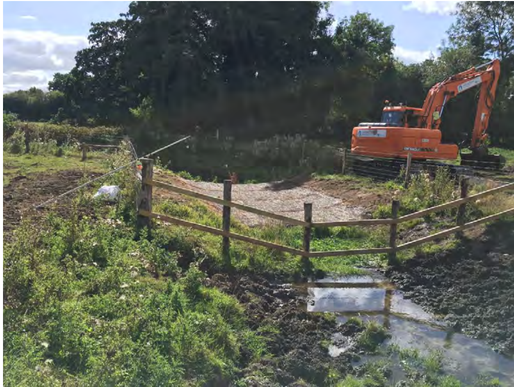
Inlet spillway with geotextile and rock roll reinforcement
