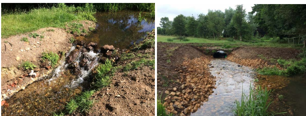
Erosion and temporary repair
