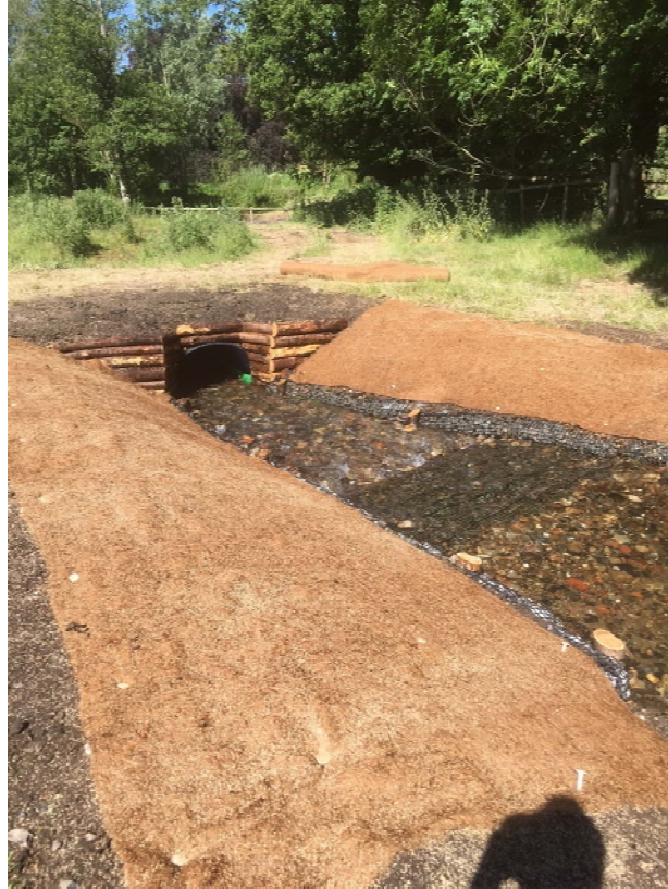
Bed, bank and erosion repairs in new bypass channel
