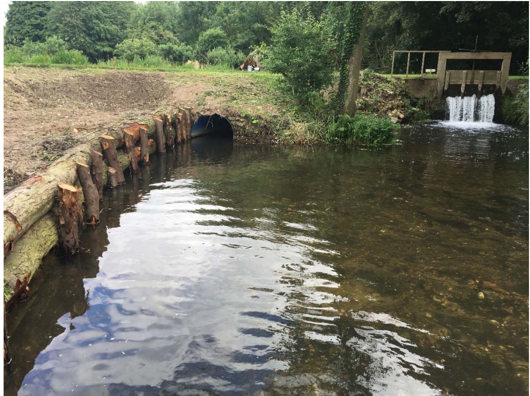
Bank erosion repairs downstream of culvert
