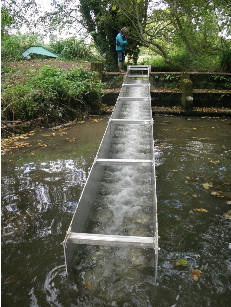
Fish and Eel pass in place
