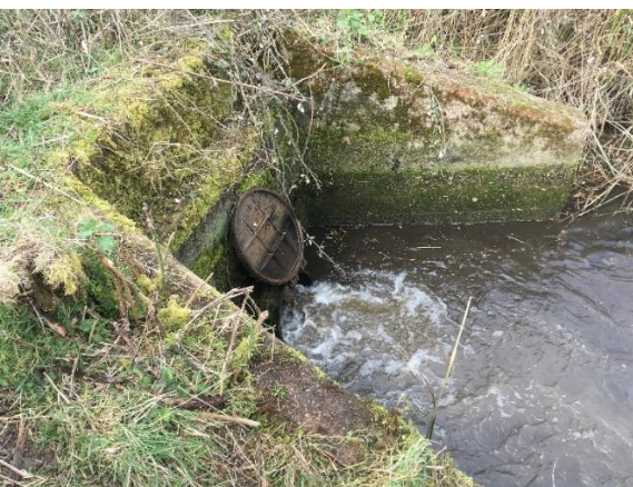
Feed Bucket (5 in total were removed) blocking the culvert and the subsequent full bore flow on removal
