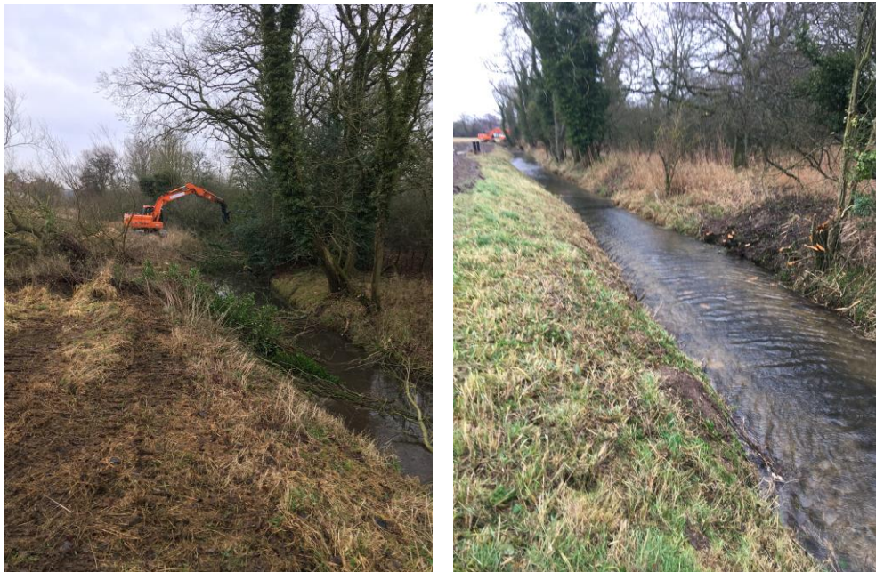
Before and after pictures on one section of watercourse. Silt sensitively removed and gravel bed now restored.
