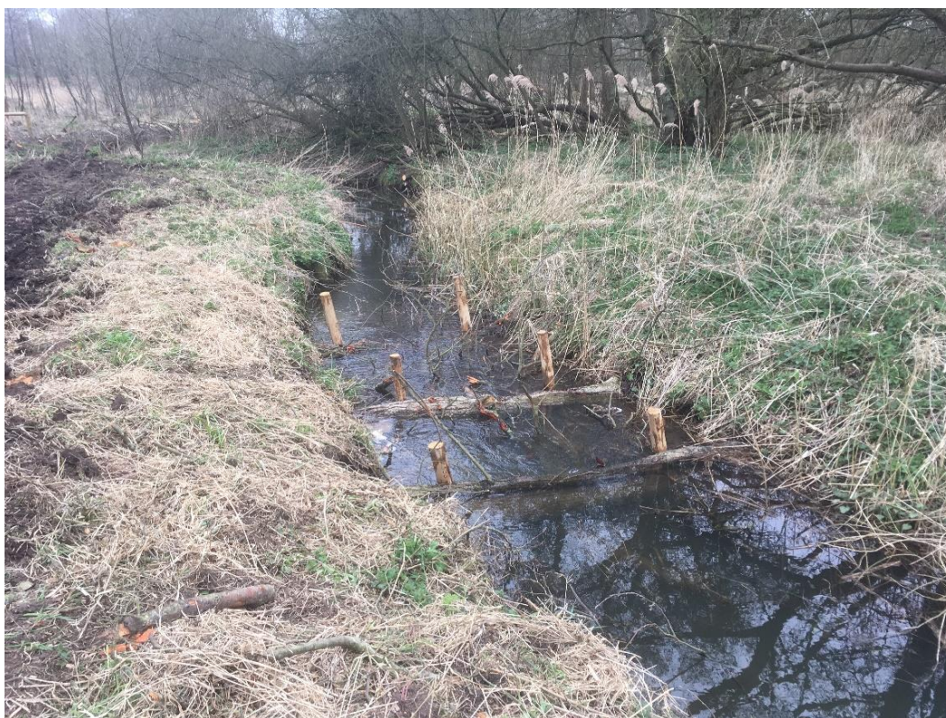
Wooden mattress structure being installed
