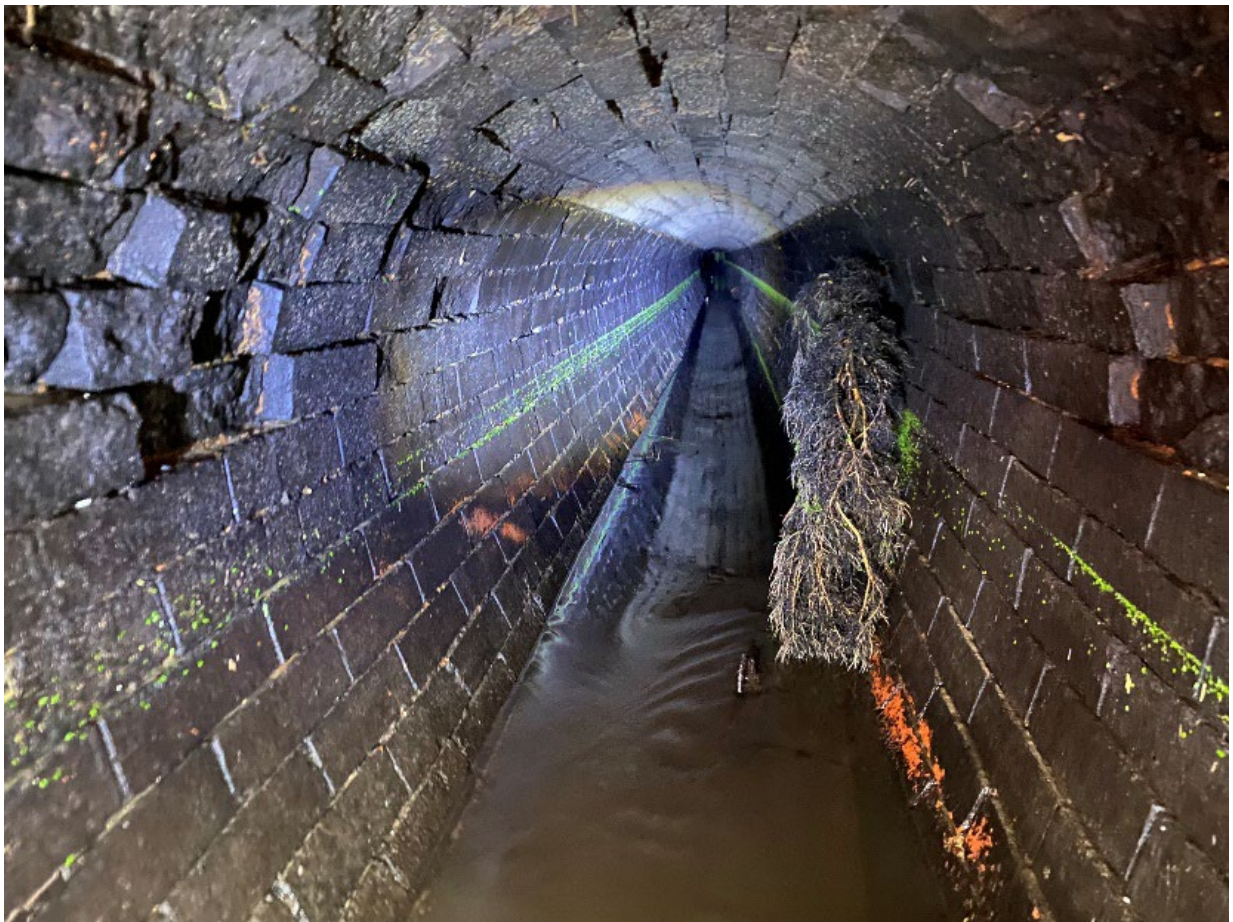
Photograph through the Elsing culvert, looking upstream.
