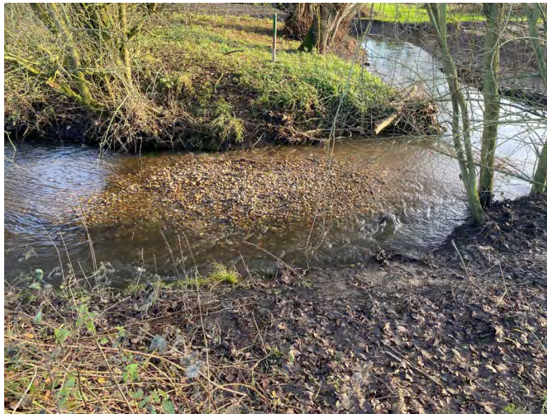
The gravel glide feature overtopping in moderate flows, showing that more gravel is required to increase it's height.
