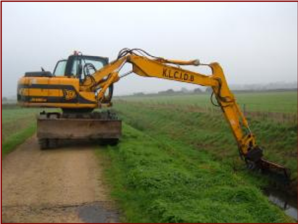
A Board's wheeled vehicle carries out desilting work on a boards main drain.
