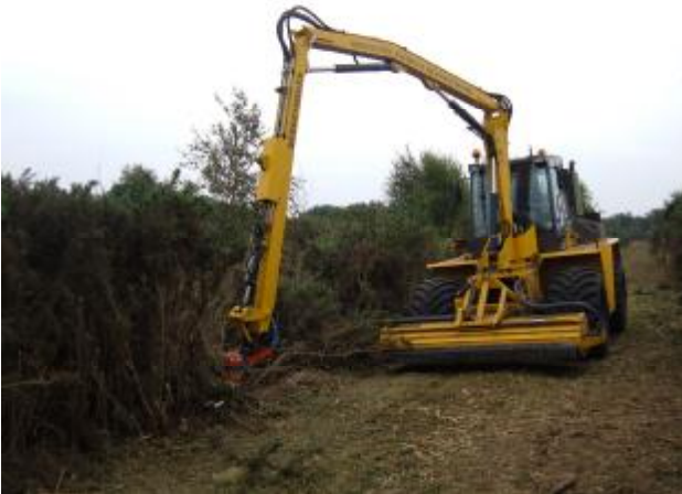
A site being cleared of gorse bushes.
