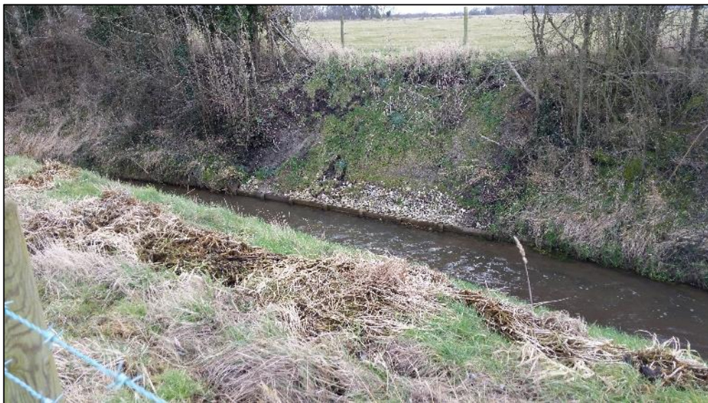
Photo 7 Showing wooden revetment on left hand bank.
