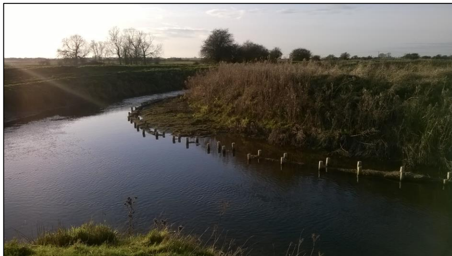
Photo 9 Previous restoration works, creating low berm.
