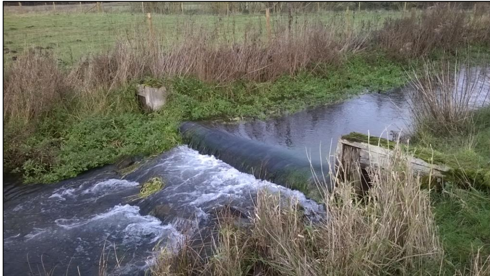
Photo 5 Small weir present through the section - propose to remove it to reduce impoundment upstream.
