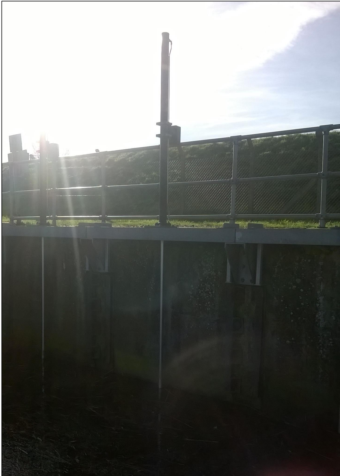
Photo 14 Babingley outfall gates
