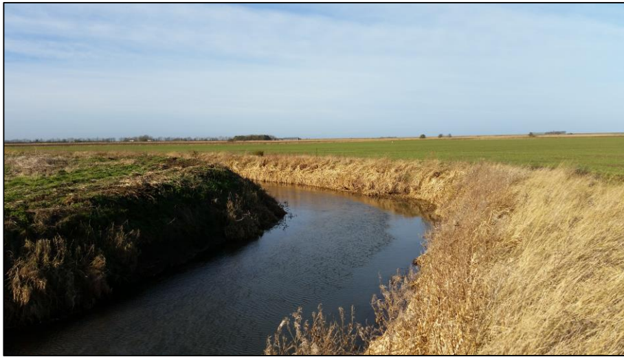
Photo 10 Wide uniform channel, wide uniform flow. Rippled surface is the result of wind.
