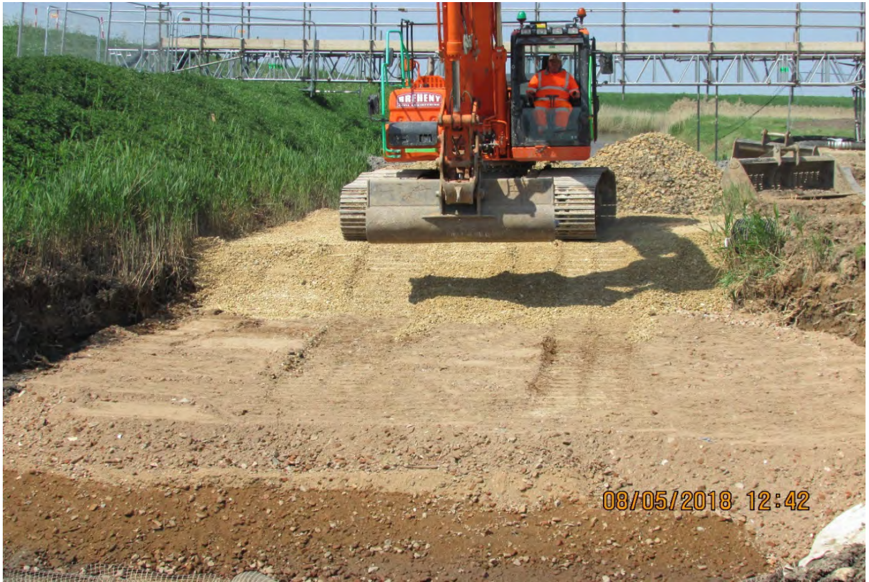
Backfilling the River Ingol
