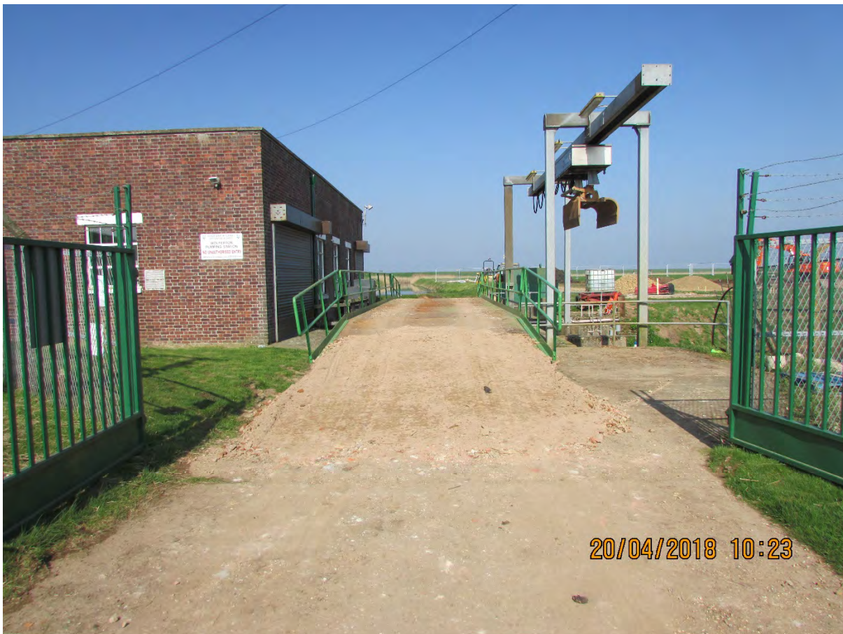
Temporary bridge to allow movement of heavy plant over the existing structure
