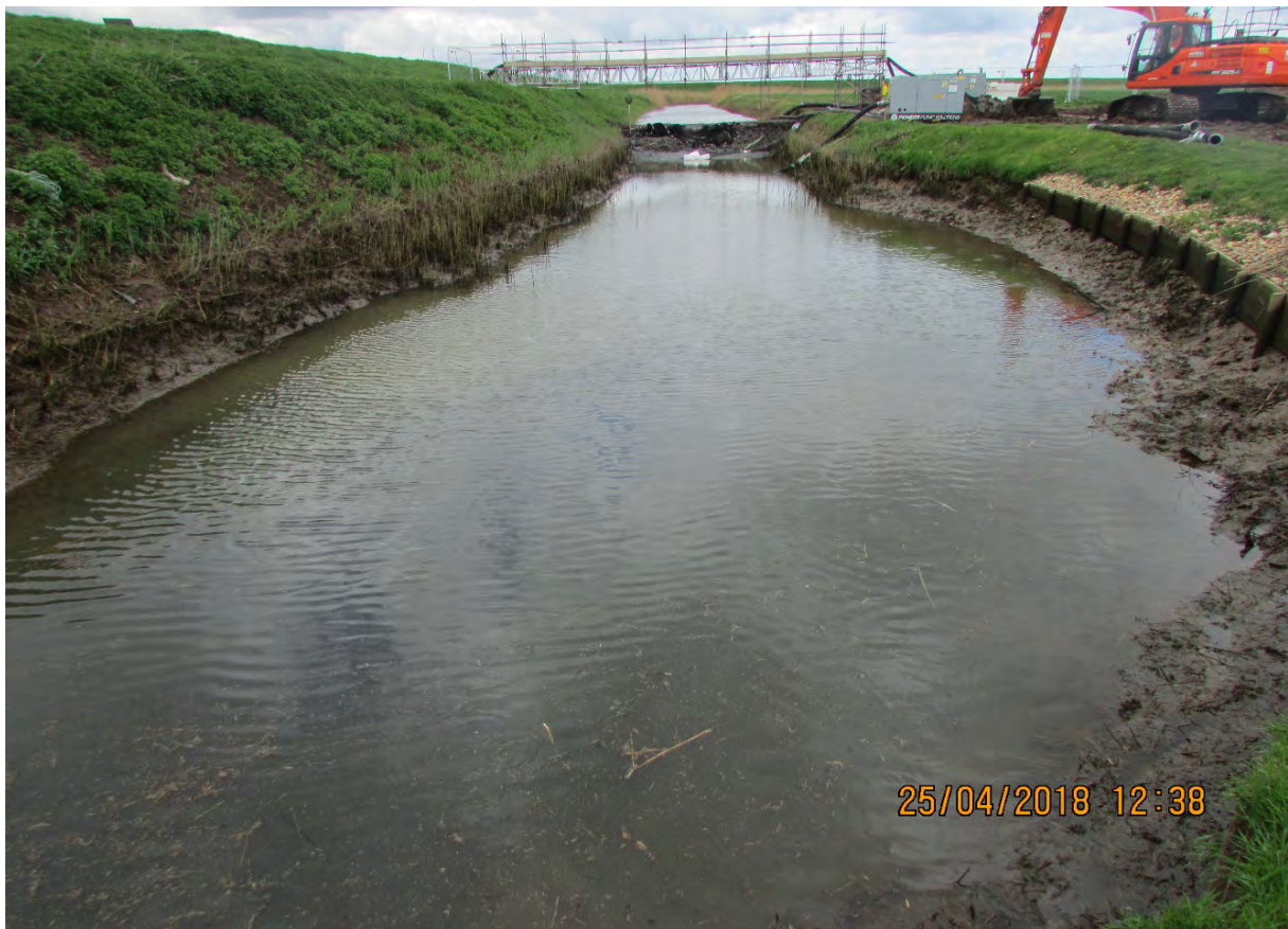
Dam and overpumping in place ready for fish rescue and backfilling. The Scaffolding in the distance forms a bridge to support the overpumping discharge pipes.
