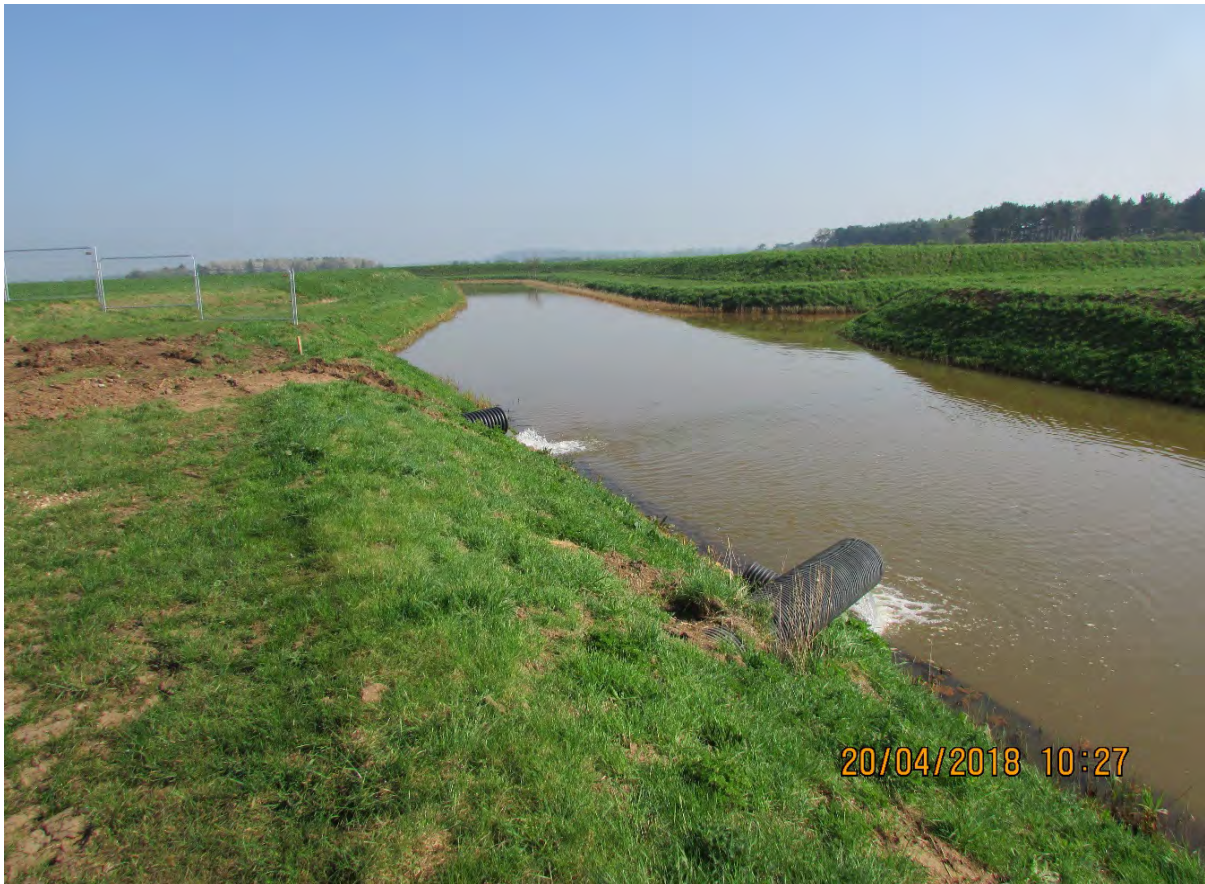
Existing, foreground (soon to be removed) and temporary overflow pipes from River Ingol
