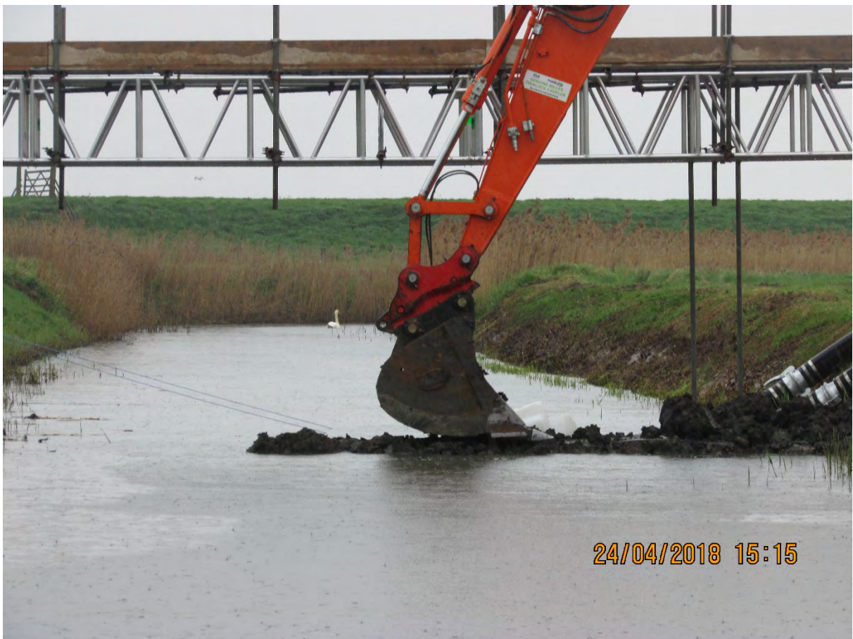
Making a start on the dam on the River Ingol
