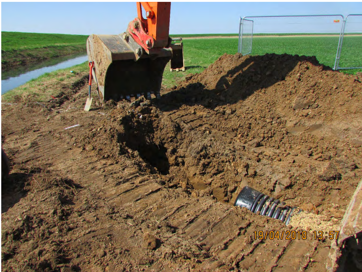
Digging the trench for the temporary overflow pipe from the River Ingol to the Boards drain to assist the overpumping during rainfall events.
