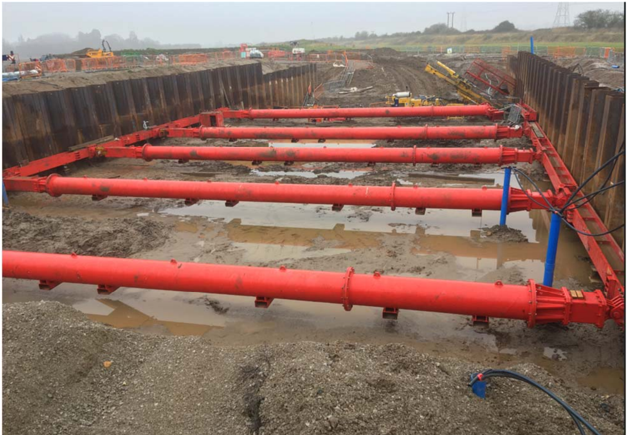
Main excavation showing temporary support frame with ground anchor rig in the background
