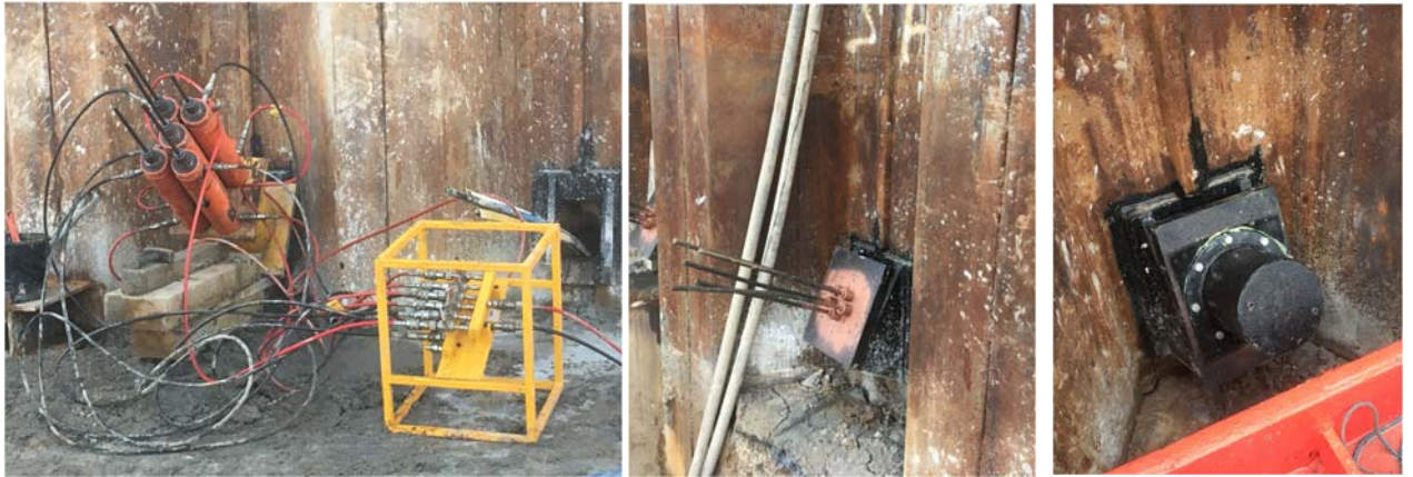
Ground anchor tendons stress loading and capped on completion
