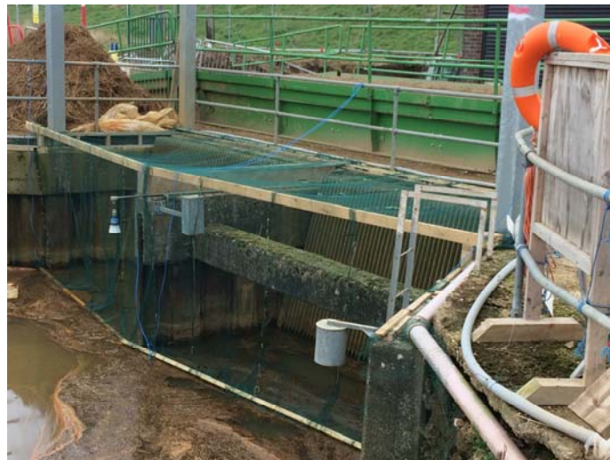
Netting in front of the pump weedscreen
