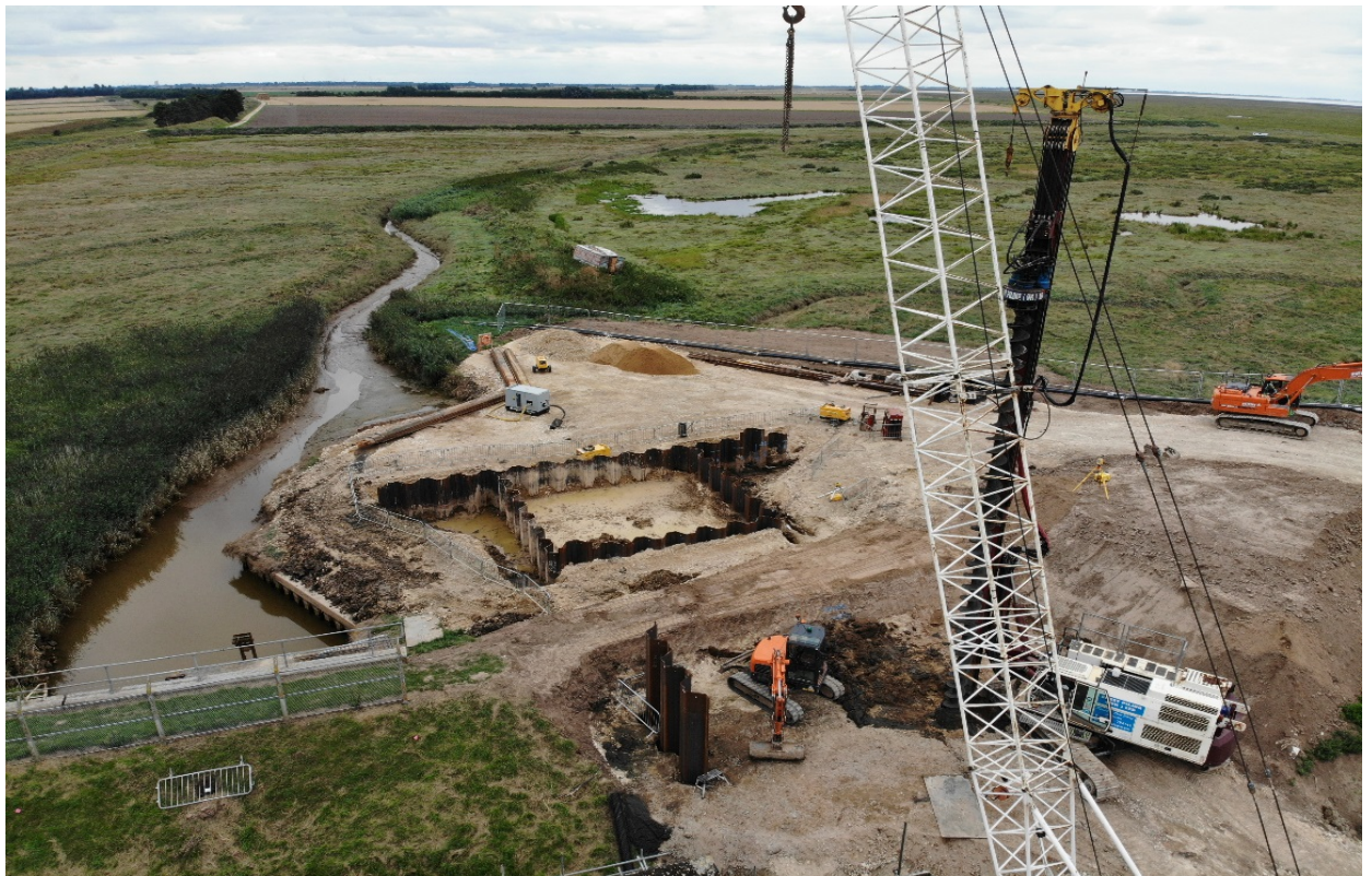
A closer view of the Outfall Structure, piling is complete and it is excavated around the outside ready for the Walings and tie rods to be installed. In the foreground you can see the Piling Rig augering ready to install the last of the piles to the Thrust Block. This view is looking over the Sea Bank.
