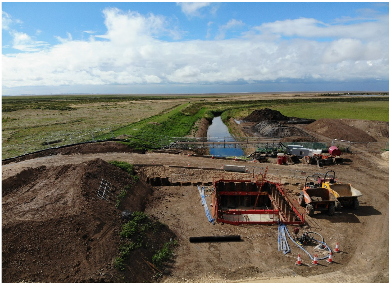
A closer view of the Ingot Intake Structure, the River can be seen in the background and is currently being over pumped.
