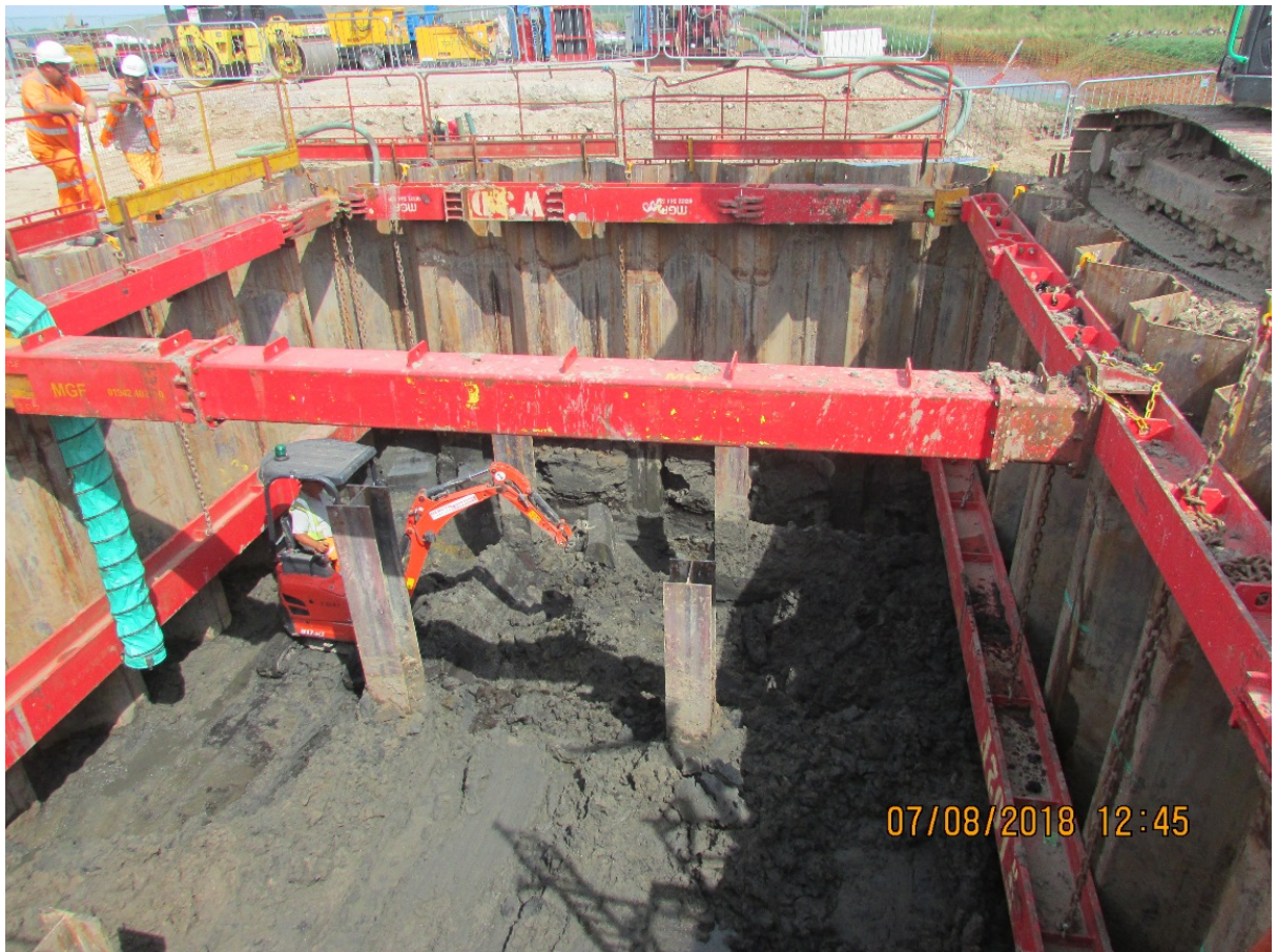
Excavation of the Pump Intake Structure. The piles protruding are required to support the weight of the dividing walls, these were hammered down to the finished dig level once excavation was complete. Due to the depth and width of the structure a mini excavator was required in the bottom to get the last of the spoil to the main excavator.
