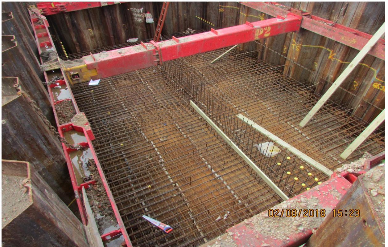
Reinforcing complete and shuttering being installed for the Ingol Intake Structure base.
