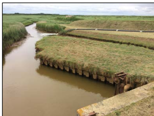
Vegetation management on the seaward side of the EA bank
