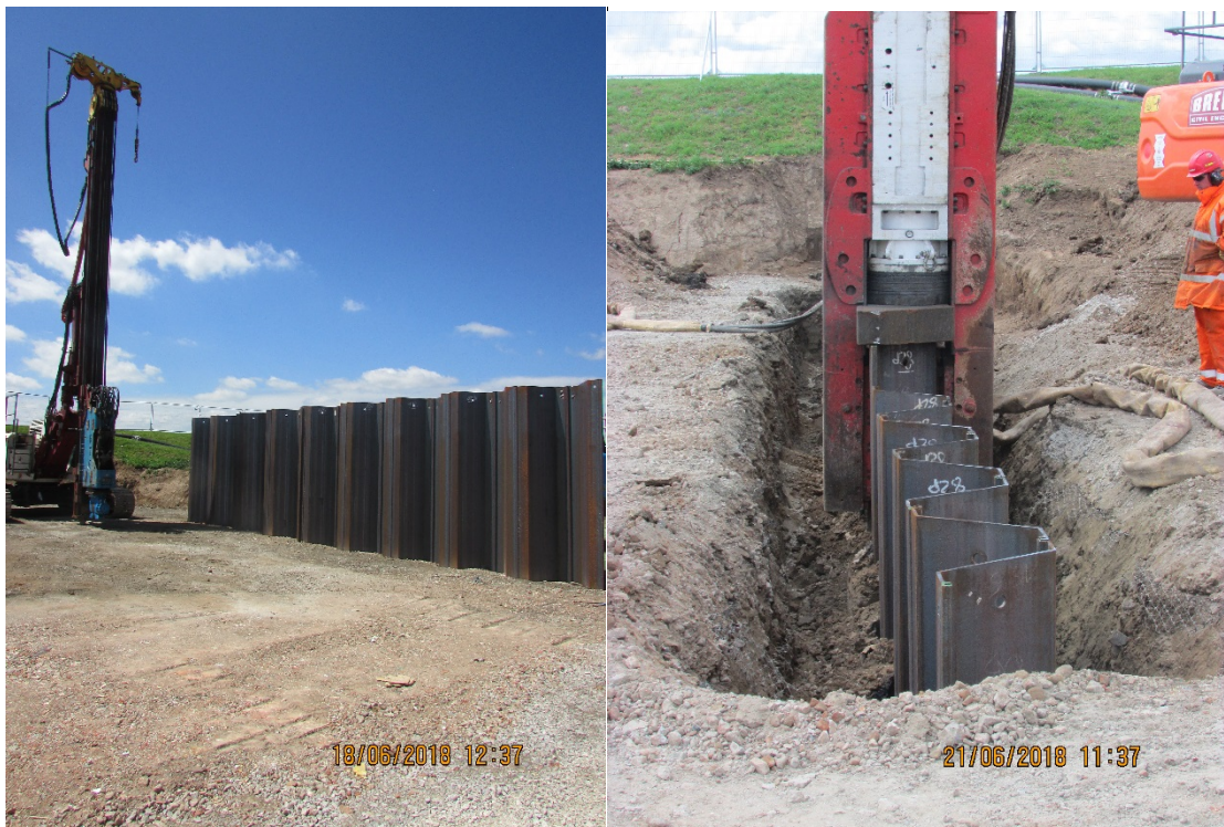
New River Ingol Inlet Structure
