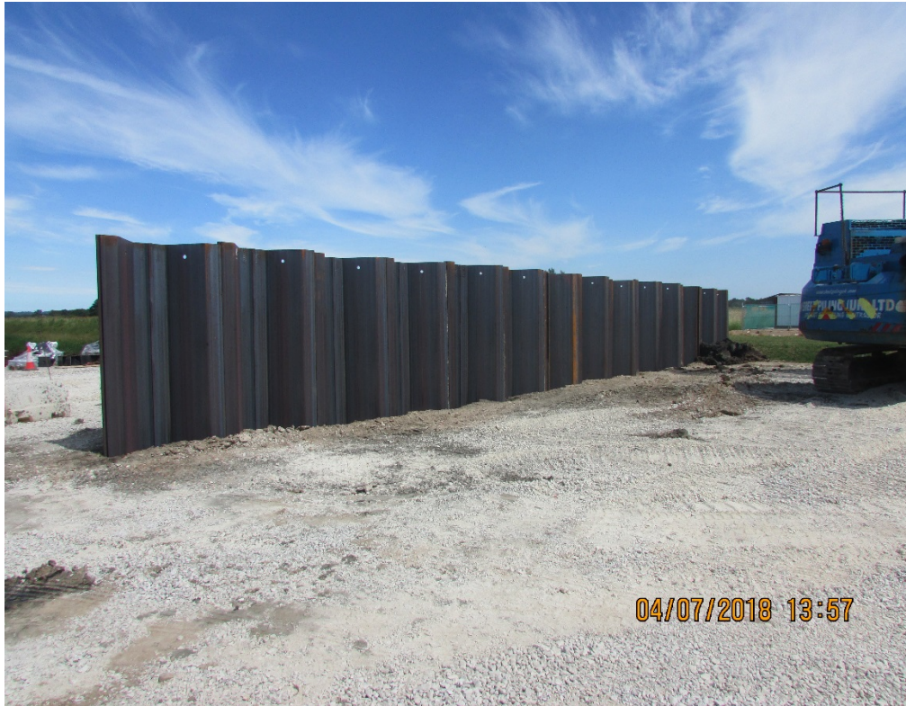
New Pumping Station Inlet Structure
