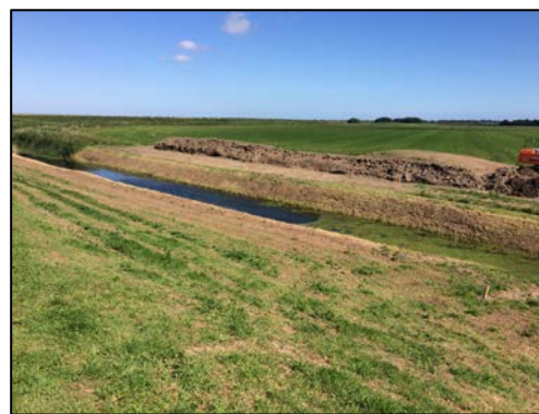
Vegetation management of the River Ingol on the landward side of the EA bank
