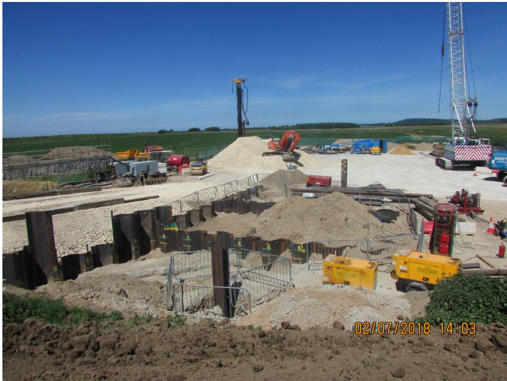
New River Ingot Inlet Structure
