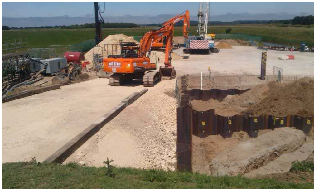
Ramp Over the Seabank
