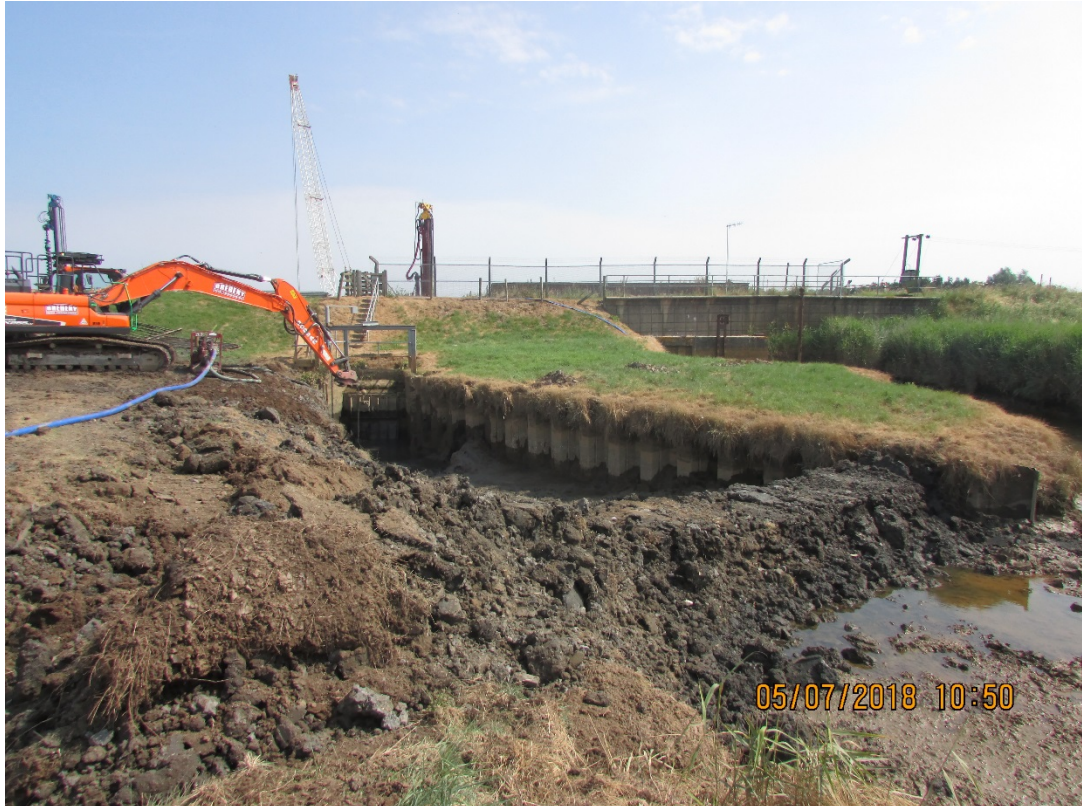
Existing River Ingol Outfall
