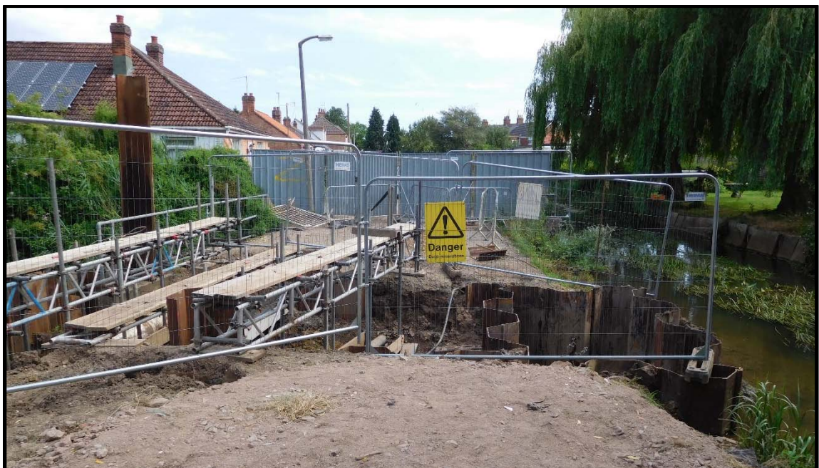
Photograph showing parts of the piling works and excavations for the new water control structure linking Gaywood River to Bawsey Drain. The scaffolding bridges are supporting various services which cross this area.
