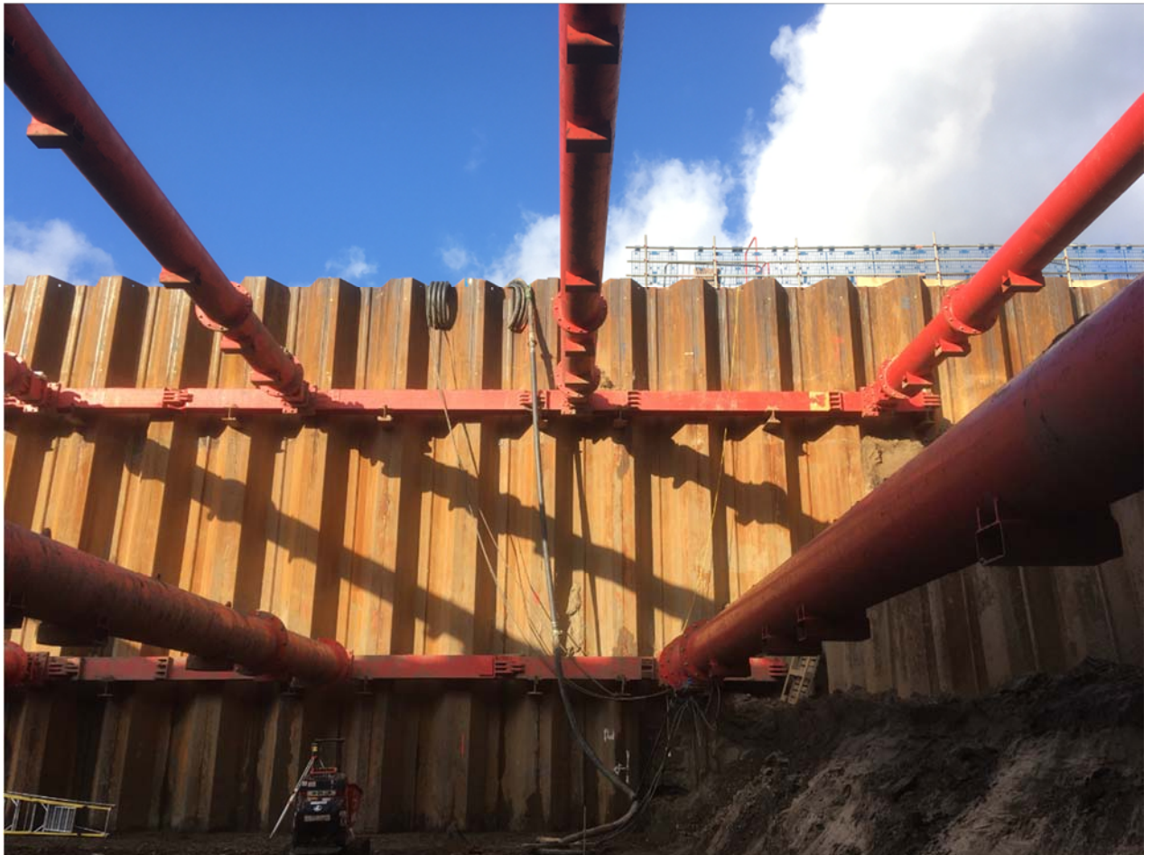
Main excavation showing temporary support frames
