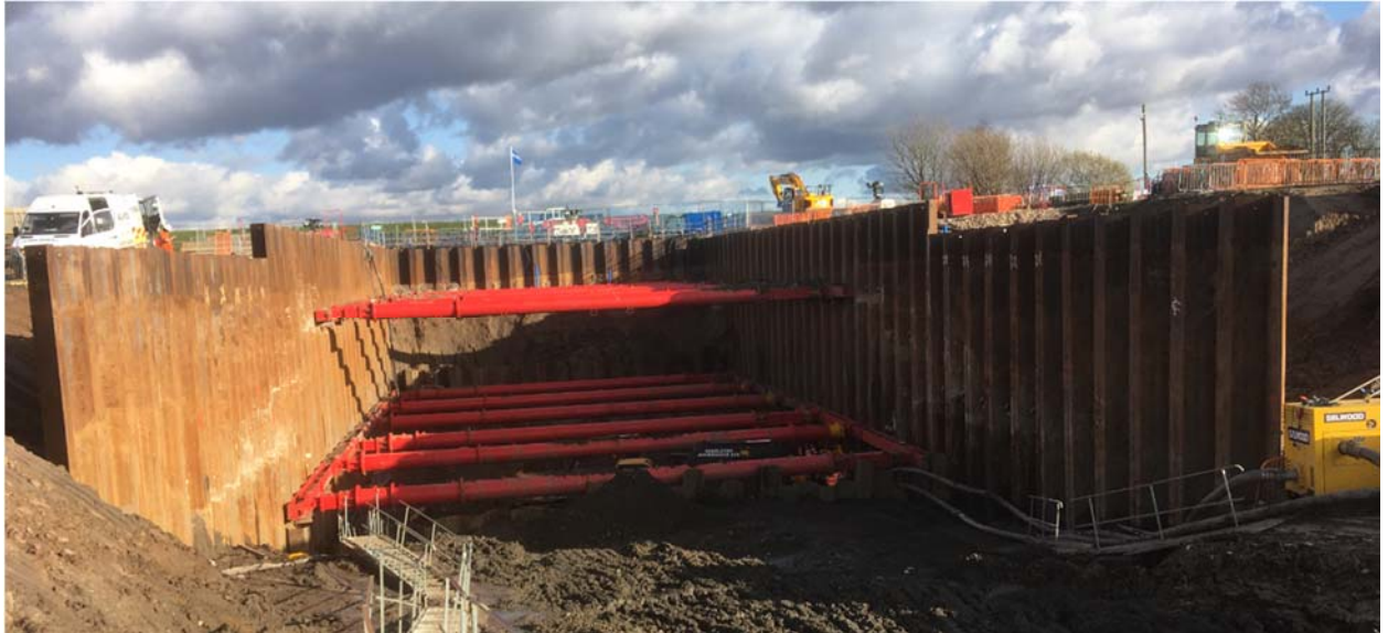
View of Cofferdam from west (intake)
