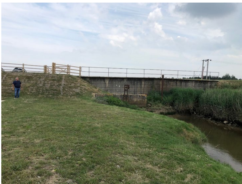
Location of seabank improvement work in front of Wolferton Pumping Station
