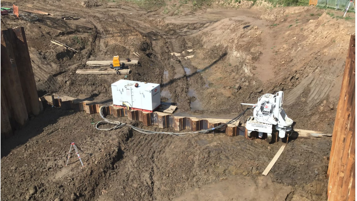
Temporary closing sheet pile wall being installed by “silent” pile press
