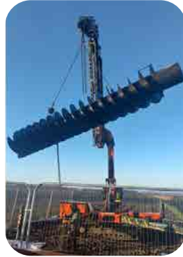
New Archimedes Screw being lifted into position in November 2025 Aerial Image of the upgraded Waltham Farm Pumping Station. Photo Credits WMA
