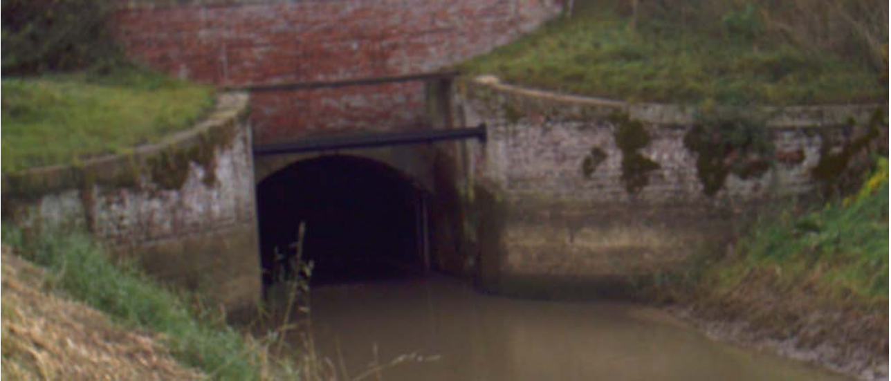
Outfall from the landward side – Straight Mile Storage Area
