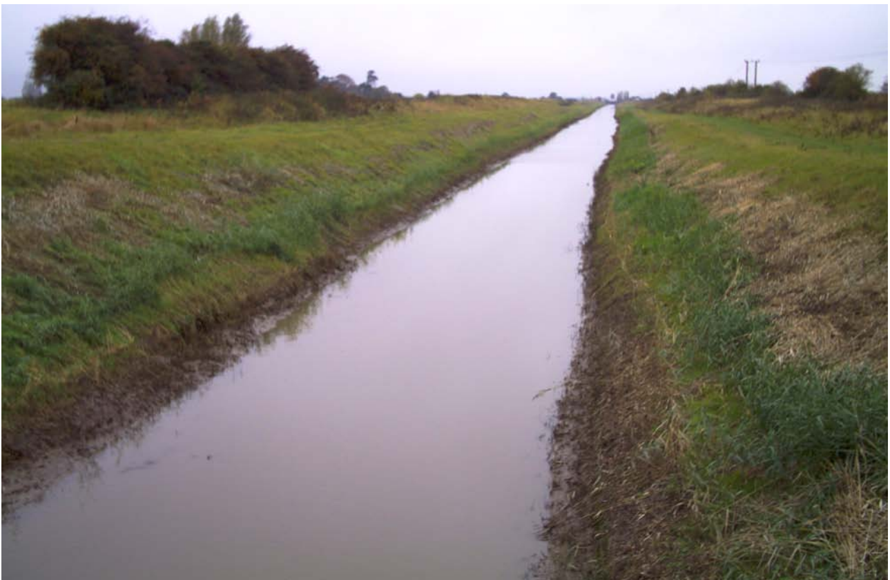
Straight Mile Storage Area – taken from outfall gates with pumping station in background
