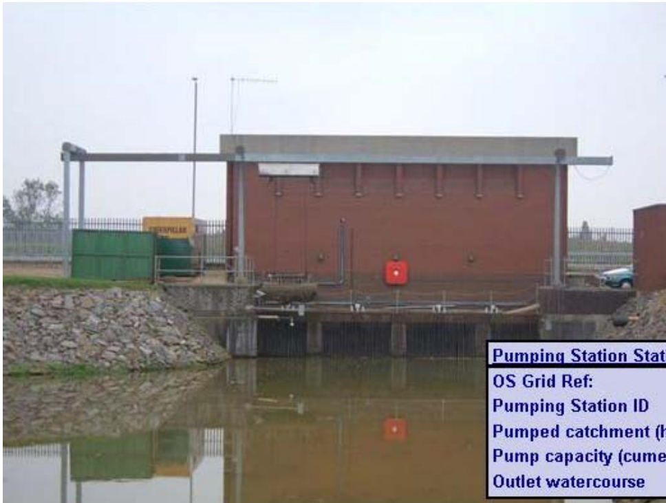
Pierrepoint Pumping Station from upstream
