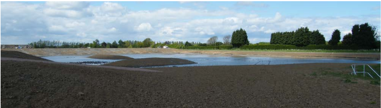
Views of Emneth Hungate Flood Storage Ponds shortly after construction
