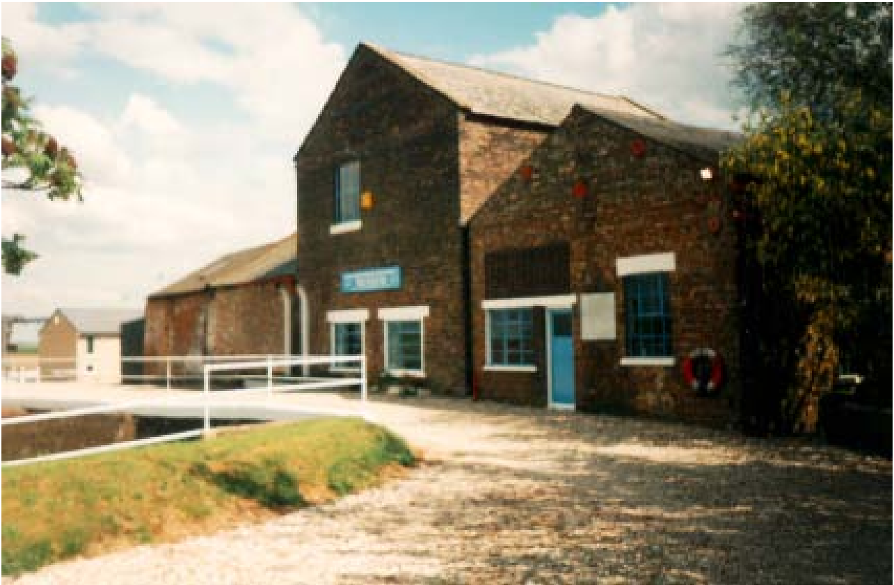
Greenbank Pumping Station and Museum (new station to the left of the picture)
